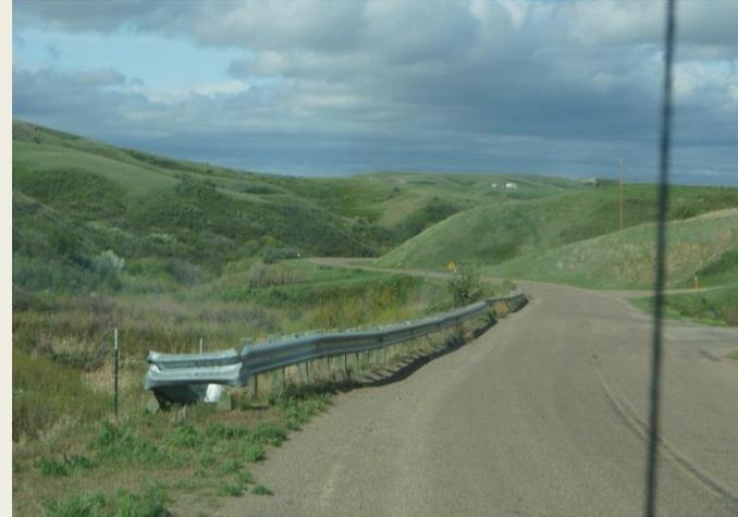
Guardrail is lacking reflective tabs and repairs
