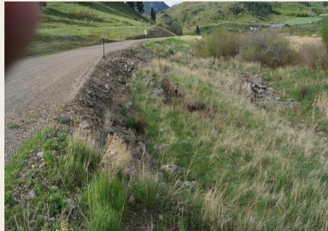
Subgrade and base failure caused rough
