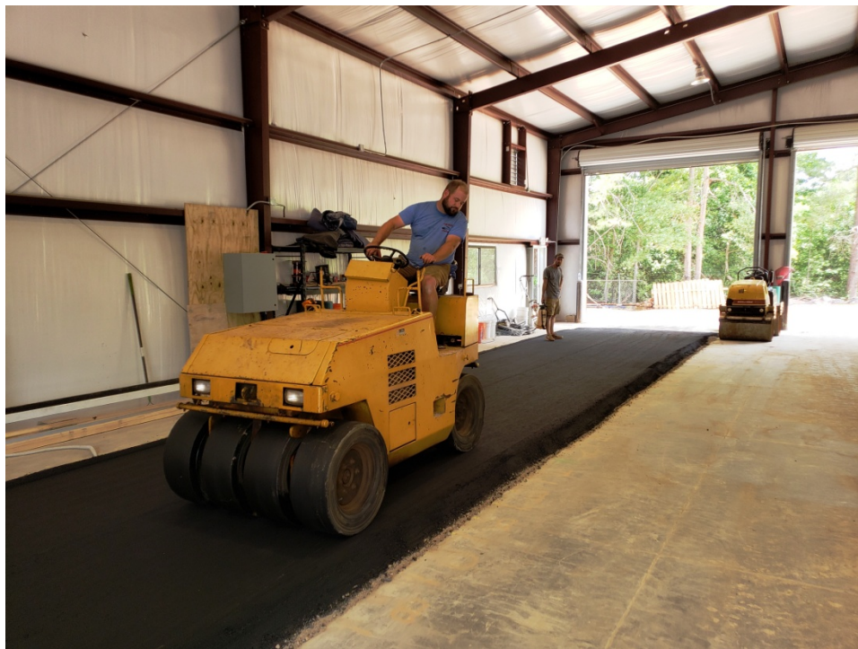
Figure 7-3: Compaction of hot-mix asphalt with a pneumatic roller.
