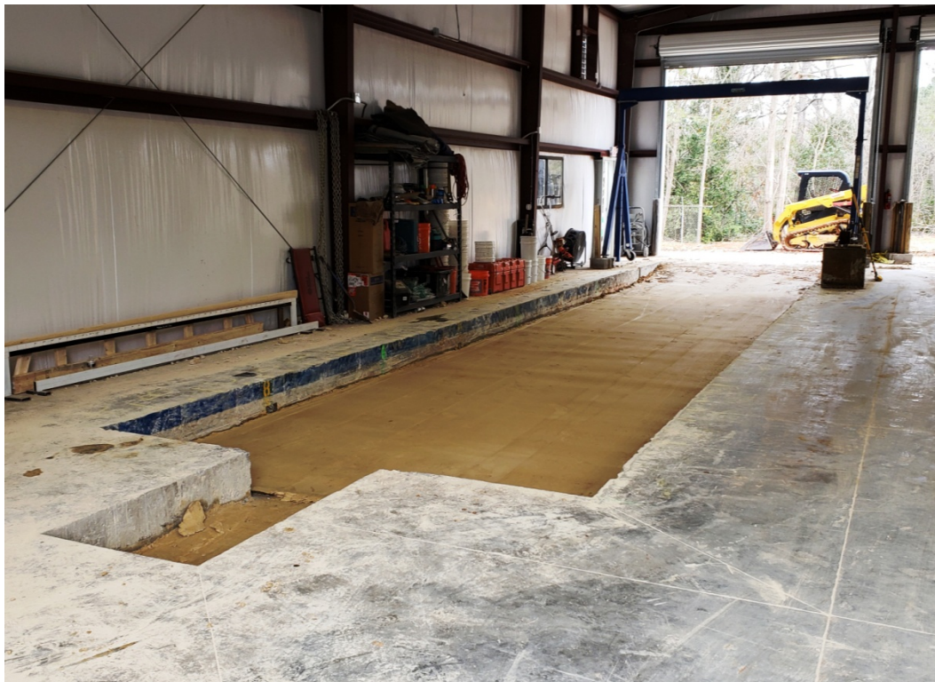
Figure 3-4: Finished surface of the subgrade.
