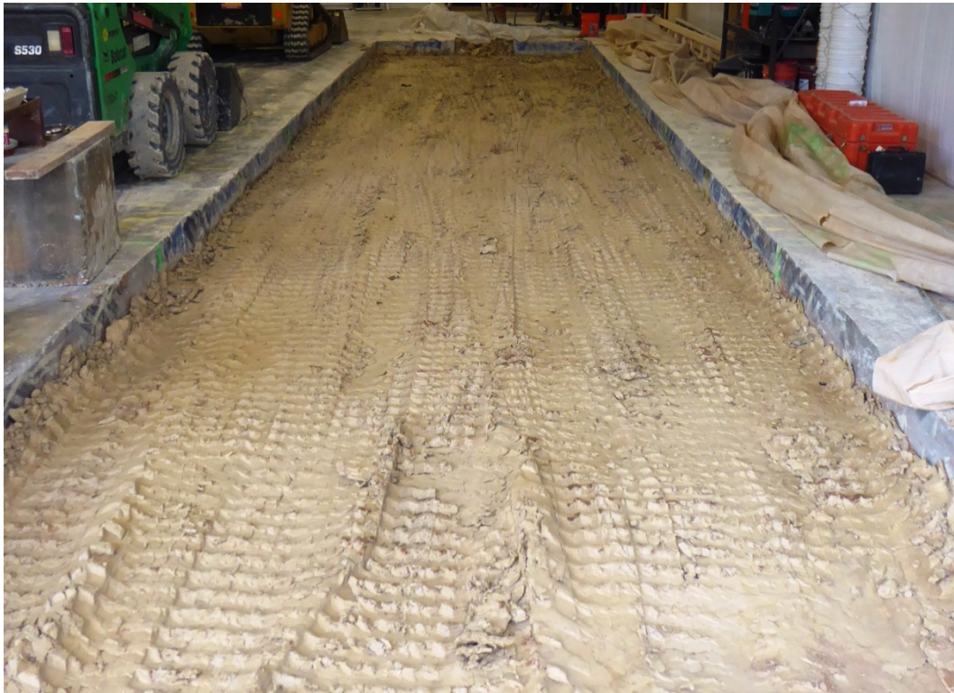
Figure 3-1: Spread and tracked subgrade prior to compaction.
