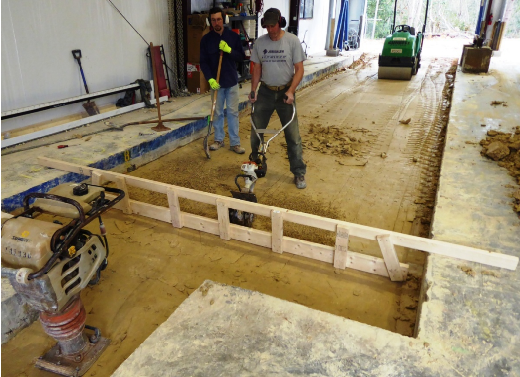
Figure 3-3: Leveling the final surface of the subgrade.
