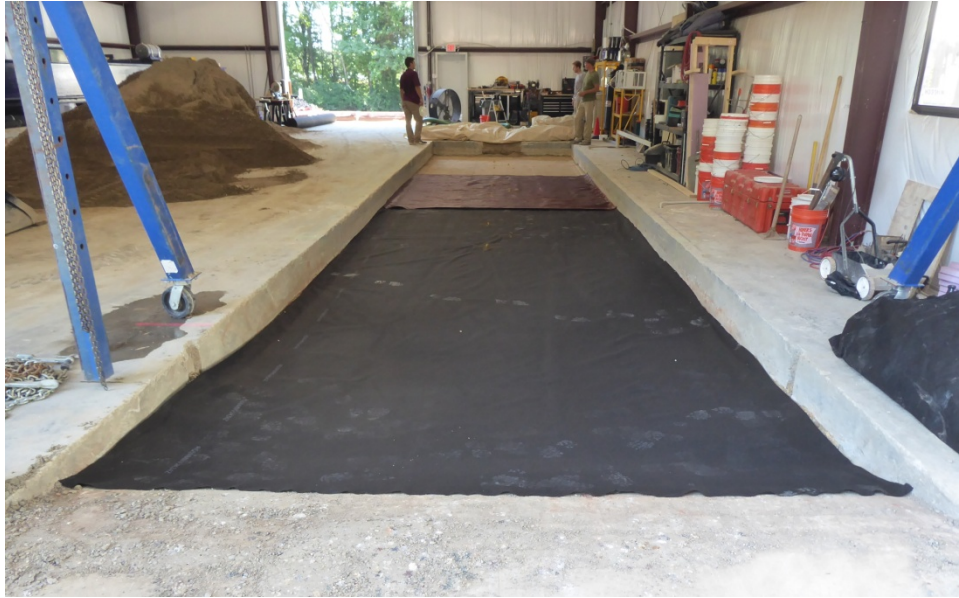
Figure 5-2: Installed geosynthetics.
