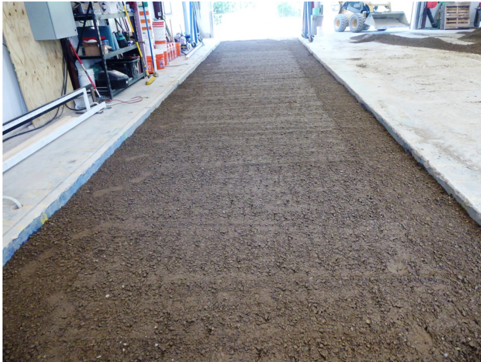
Figure 6-1: First layer of gravel screed to uniform depth.
