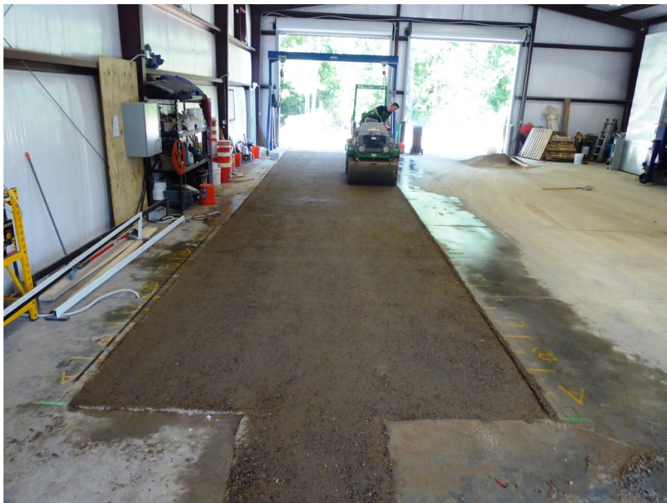
Figure 6-2: Final compacted surface of the base course.
