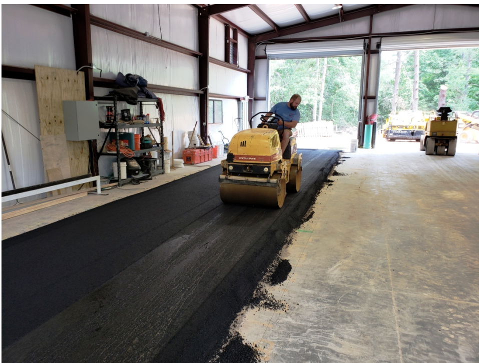
Figure 7-2: Compaction of hot-mix asphalt using a smooth drum roller.
