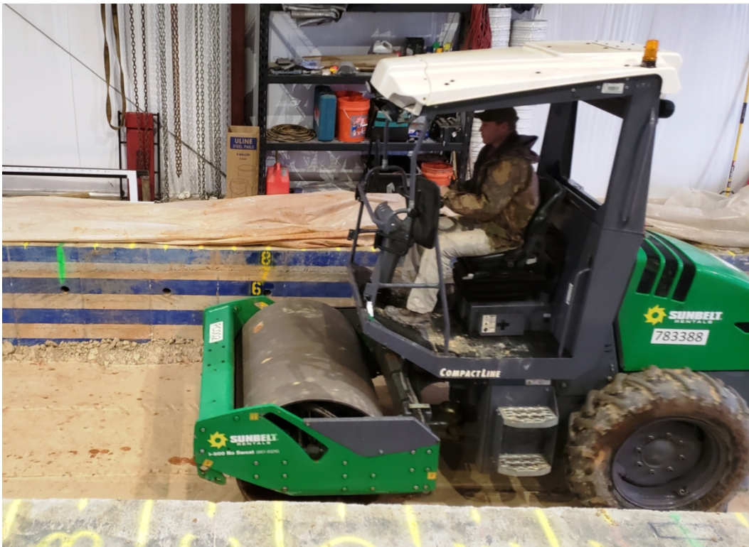
Figure 3-2: Compacting the subgrade.
