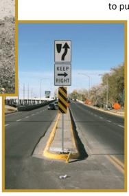
Since the original installation in 2012, several units have been struck and performed as advertised, with the signs being re-installed in about 10 minutes.
