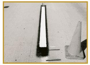
durability with snow plow use. The increased retroreflectivity during wet conditions is also being evaluated to determine their effectiveness as safety treatments.
