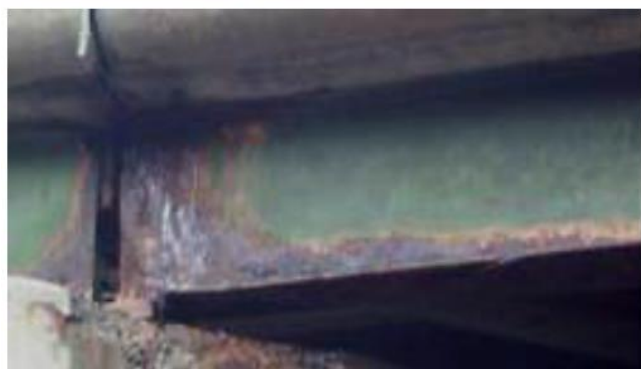
a) Typical end corrosion of bridge girders
