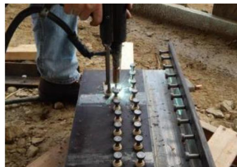
b) Installation of shear studs for UHPC repair
