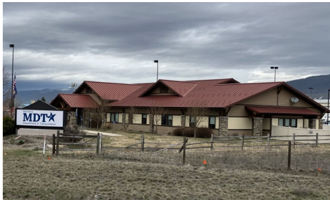
New Missoula District Headquarters building.
