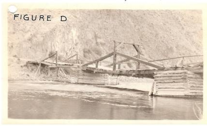
Browne's Bridge as it appeared after being condemned by the counties in 1915 due to severe structural damage from a fire.
