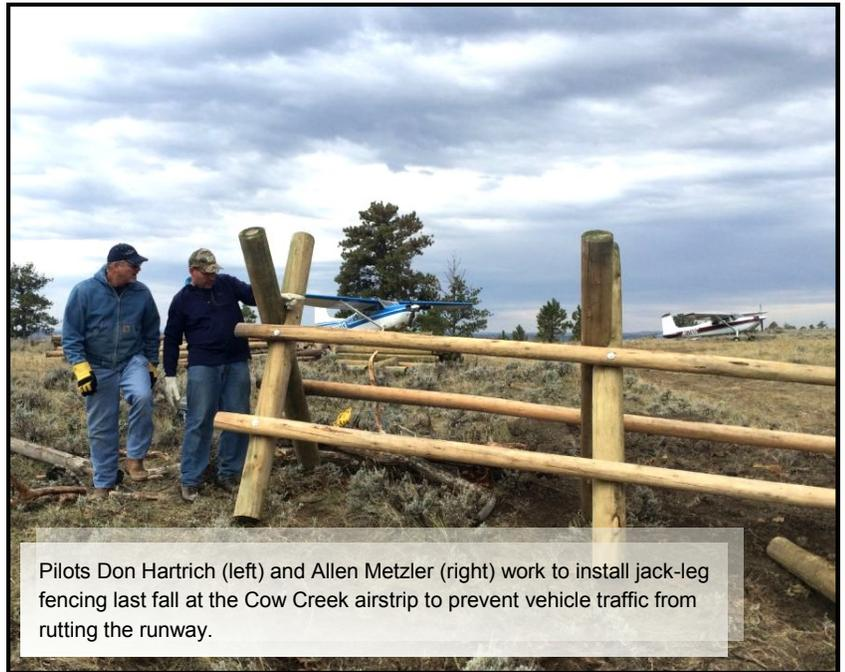
Pilots Don Hartrich (left) and Allen Metzler (right) work to install jack-leg fencing last fall at the Cow Creek airstrip to prevent vehicle traffic from rutting the runway.
