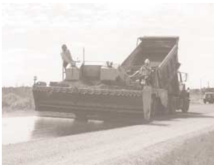
Preventive maintenance treatments, such as the chip seal shown here, can preserve the roadway and retard future deterioration.
