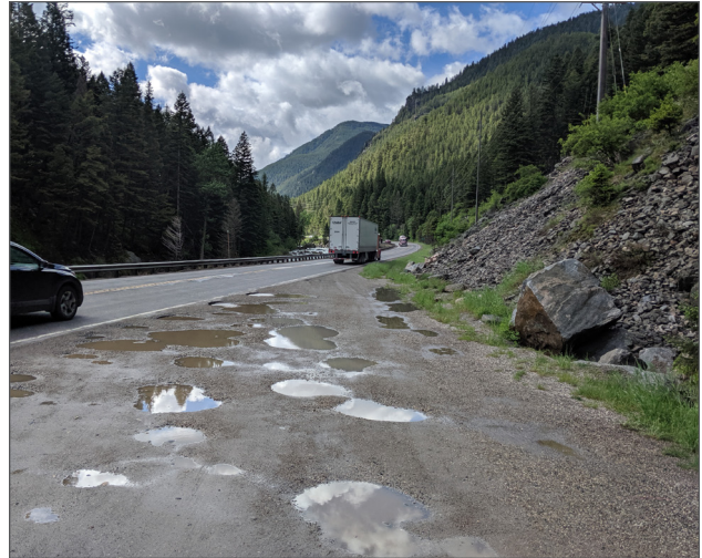
Some of the unpaved turnouts have poor drainage conditions. There are also several locations with potential for rockfall events.
