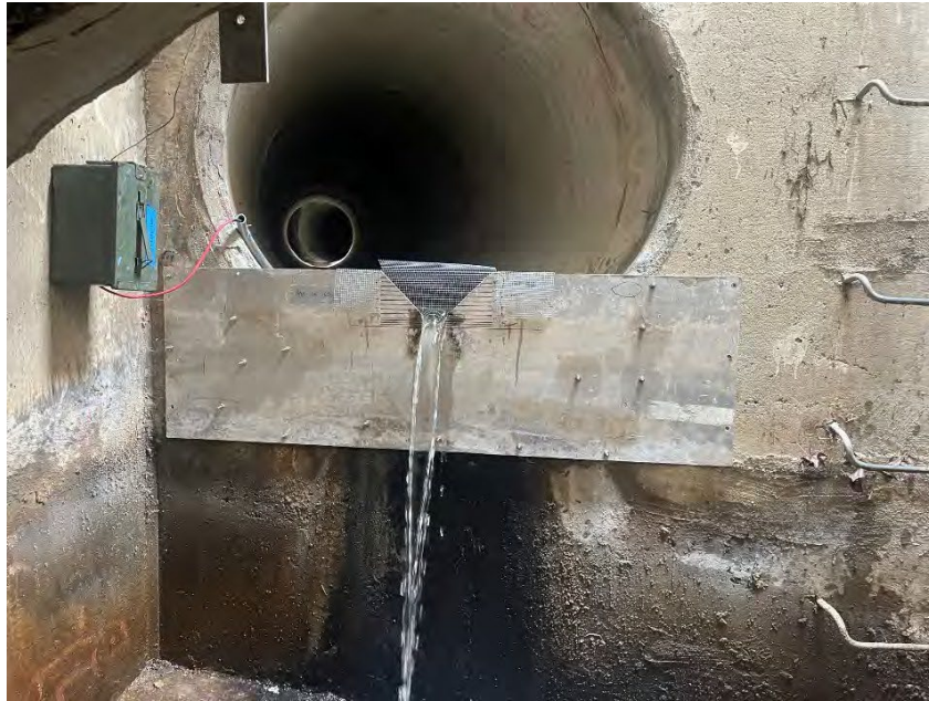
Figure 4-2. V-notch Weir on Outfall
