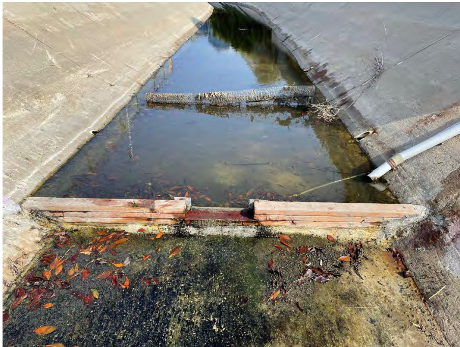
Figure 4-3. Rectangular Weir
