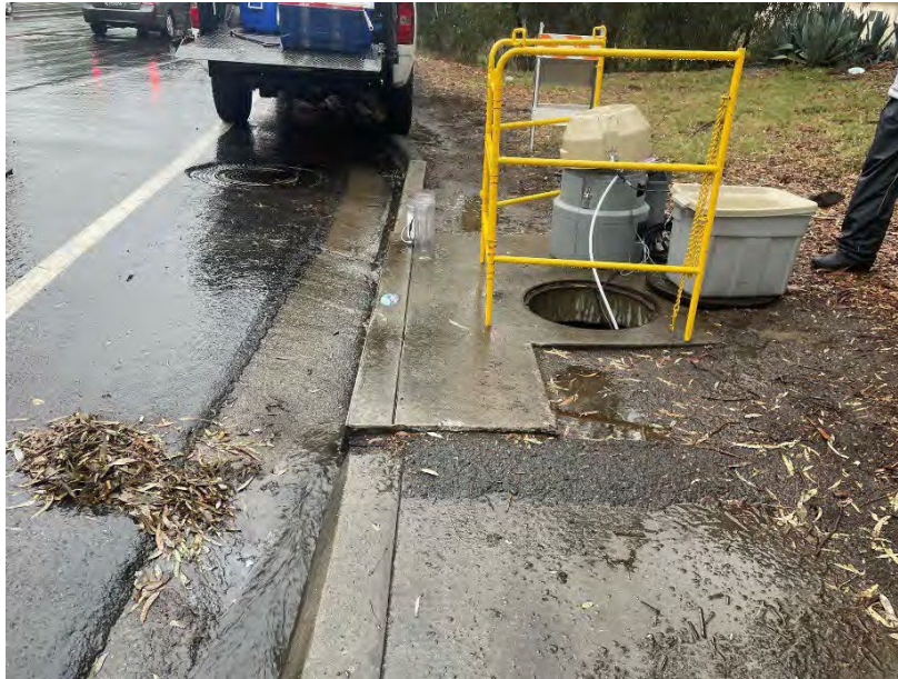
Figure 4-8b. Example of Temporary Automated Sampler Setup
