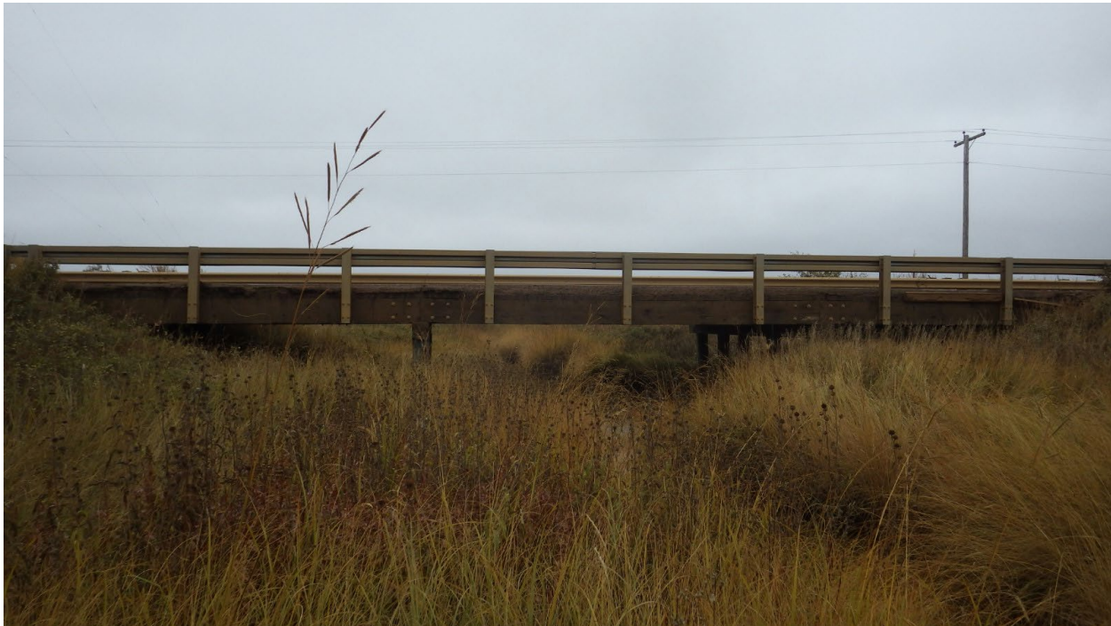
Bridge over Sandstone Creek NBI: P00027035+08231 / MDT Structure # 05697
