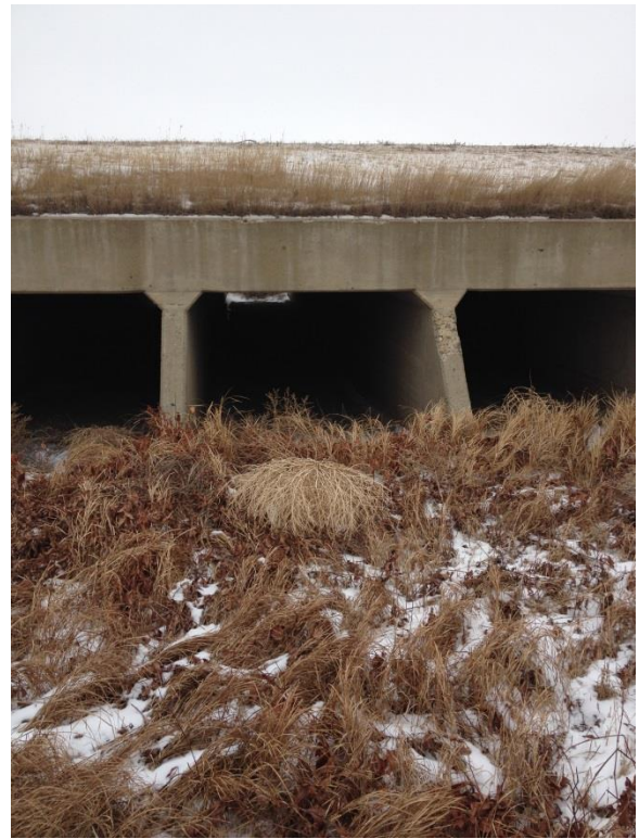
RM 13.292, Station 697+05 3-7 X 5, Box Culvert, South Side (Outlet)
