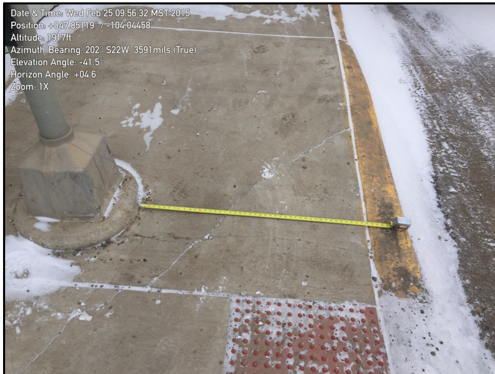
Photo 106. Looking at the southeast corner of MT 200 and 6 th Street at a signal pole that is blocking the ADA ramp. RP 63.3.
