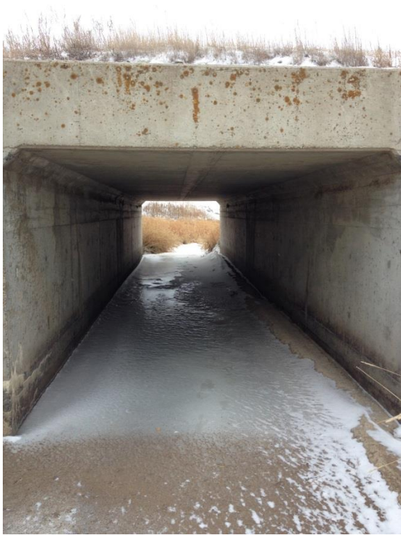
RM 1.278, Station 67+49 10 X 10 Box Culvert – North Side (Outlet)
