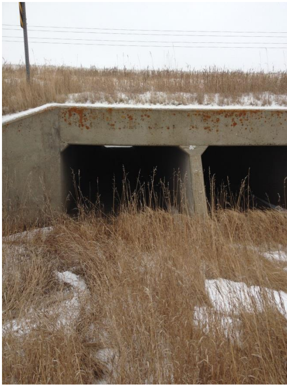
RM 13.292, Station 697+05 3-7 X 5, Box Culvert, North Side (Inlet)
