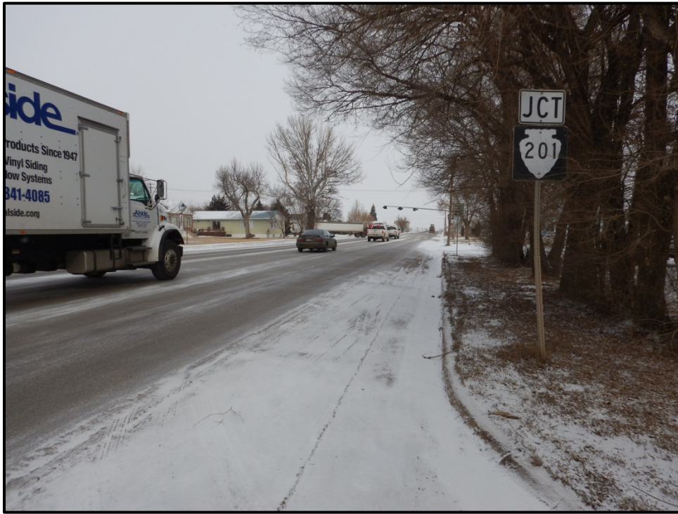
Photo 114. Looking north on MT 200. The sidewalk on the southeast side of the roadway discontinues at this point, approximately one block south of the city park. RP 63.6.
