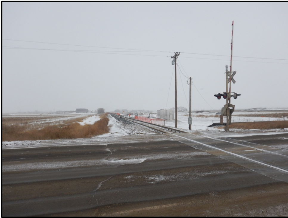
Photo 126. Looking north on ND 200 at a railroad crossing. Roadway rutting is more severe in this location compared to other locations within the study area. RP 0.1.
