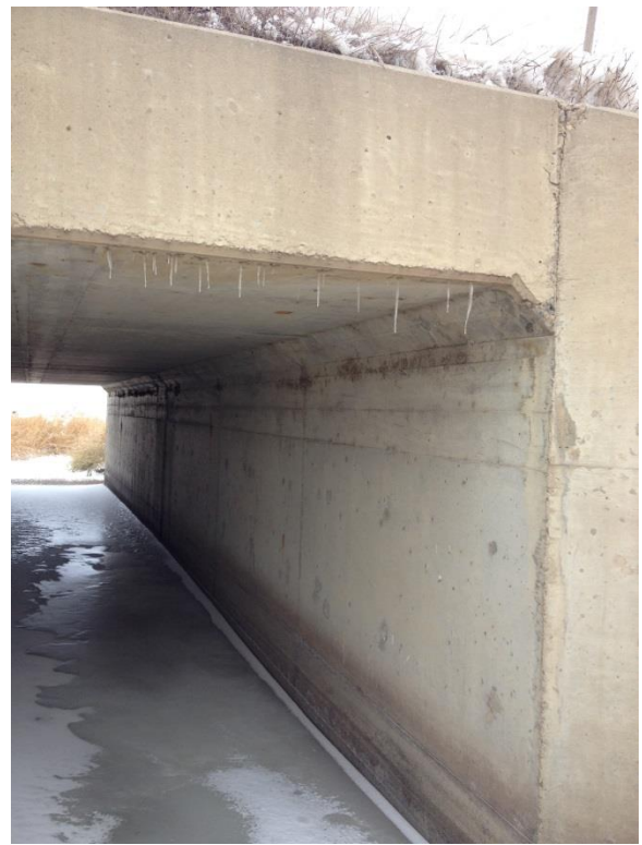
RM 1.278, Station 67+49 10 X 10 Box Culvert – South Side (Inlet)
