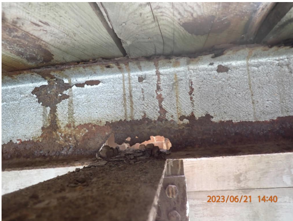
Photo 2: Stringer 8 at Floorbeam 2
