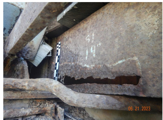
Photo 3: Stringer 1 at Abutment 2
