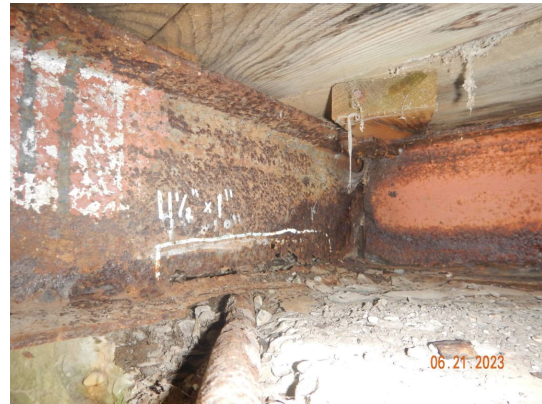
Photo 1: Stringer 8 at Abutment 1
