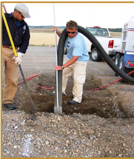
Figure 3. Air and vacuum removal of base course during forensic investigations.
