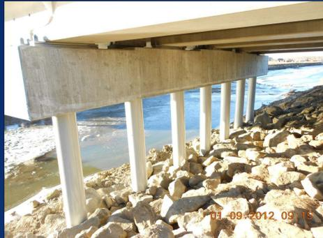
Typical MDT Concrete-Filled Steel Pile and Concrete Pile Cap Bridge Substructure
