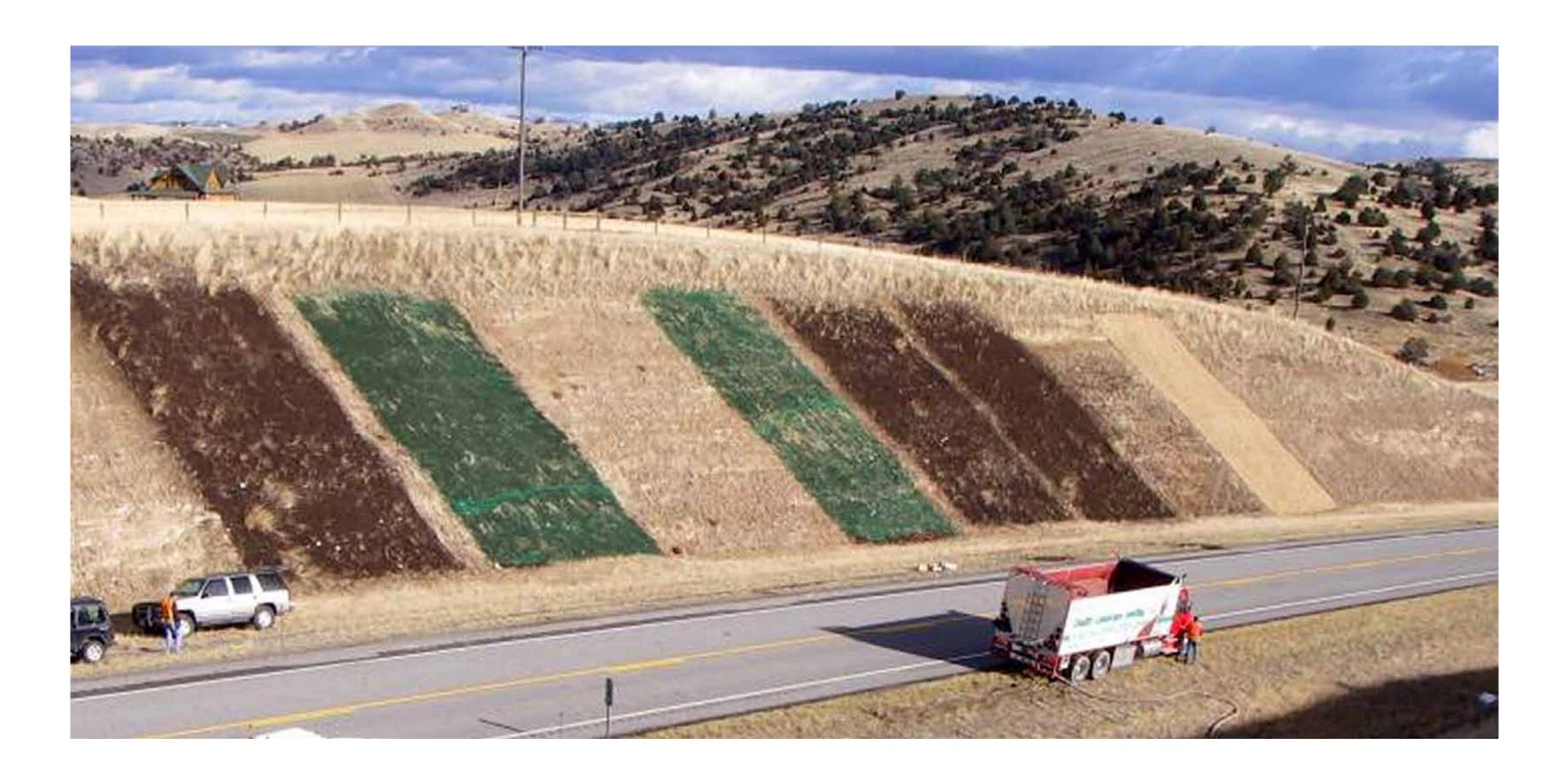
Figure 4: View of eight south-facing plots receiving varying depths of compost and/or a compost retention treatment. Note the green plots are the plastic netting and the plot furthest to the right (east) received erosion control fabric.
