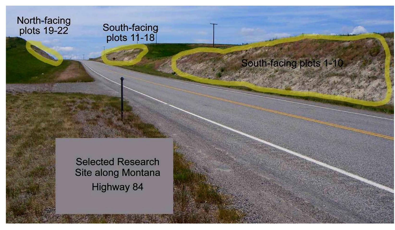
Figure 2: Roadside overview of research site location along Montana Highway 84. The slopes, 2 H:1 V, had been seeded in 2004 following reconstruction of this section of highway with minimal success of native vegetative cover.
