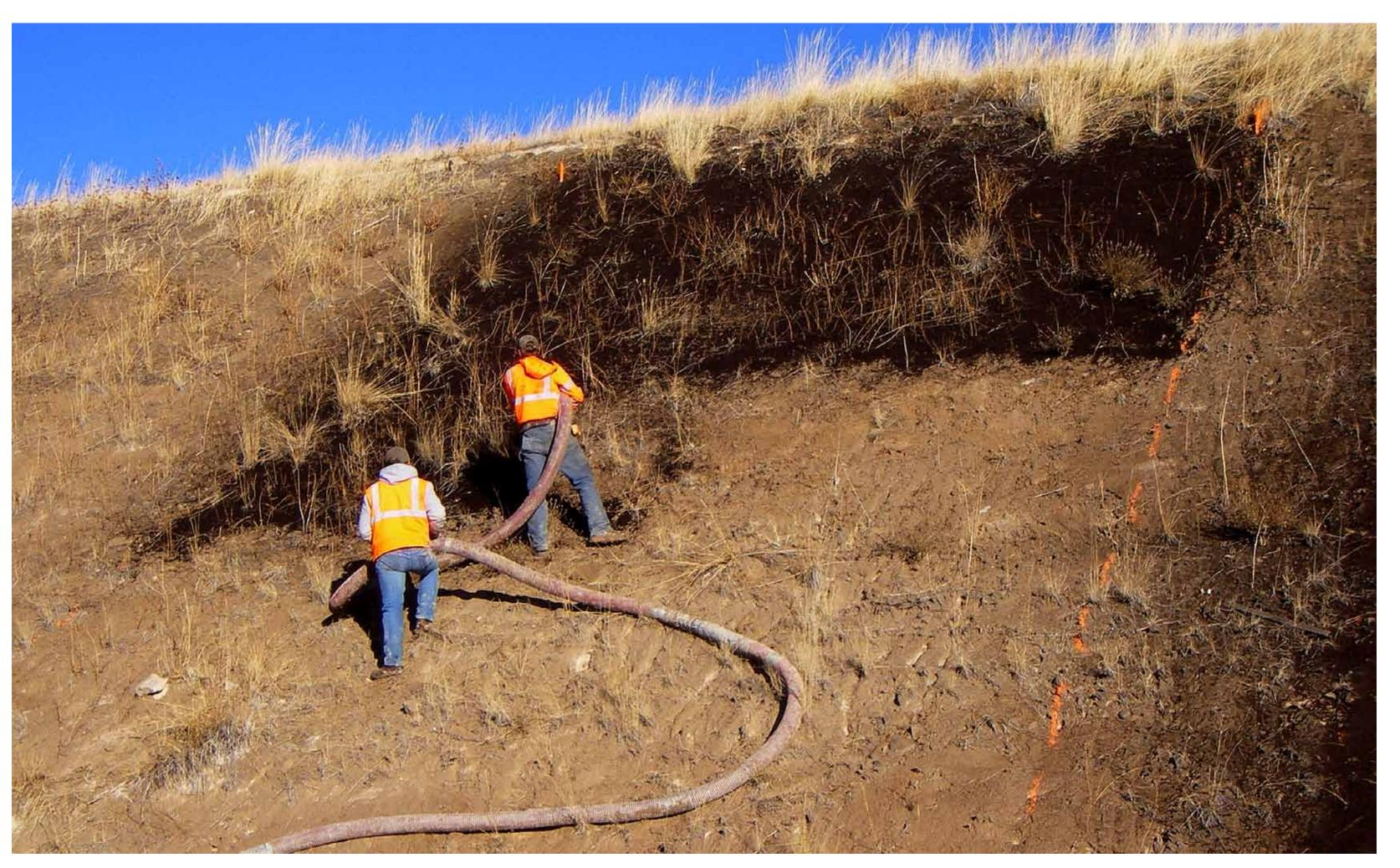
Figure 3: Application of compost on a test plot using a blower truck.
