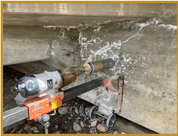
Figure 2: Coring of Backwall on Belt Creek Bridge
