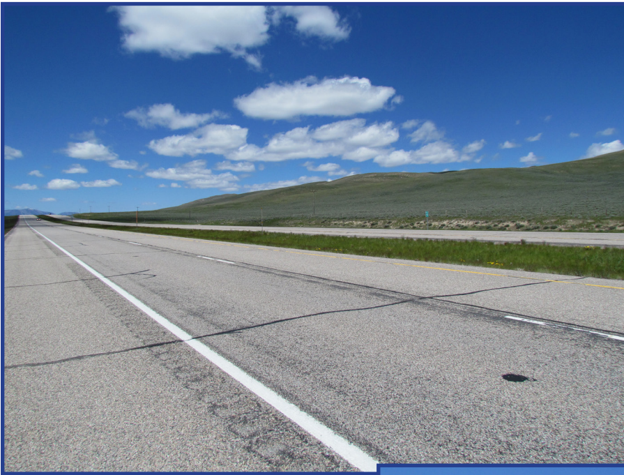
Figures 25 and 26- WMA treatment southbound (top) shows cracking near the centerline and missing seal and cover material and HMA northbound (right) exhibits similar conditions near RP 5
