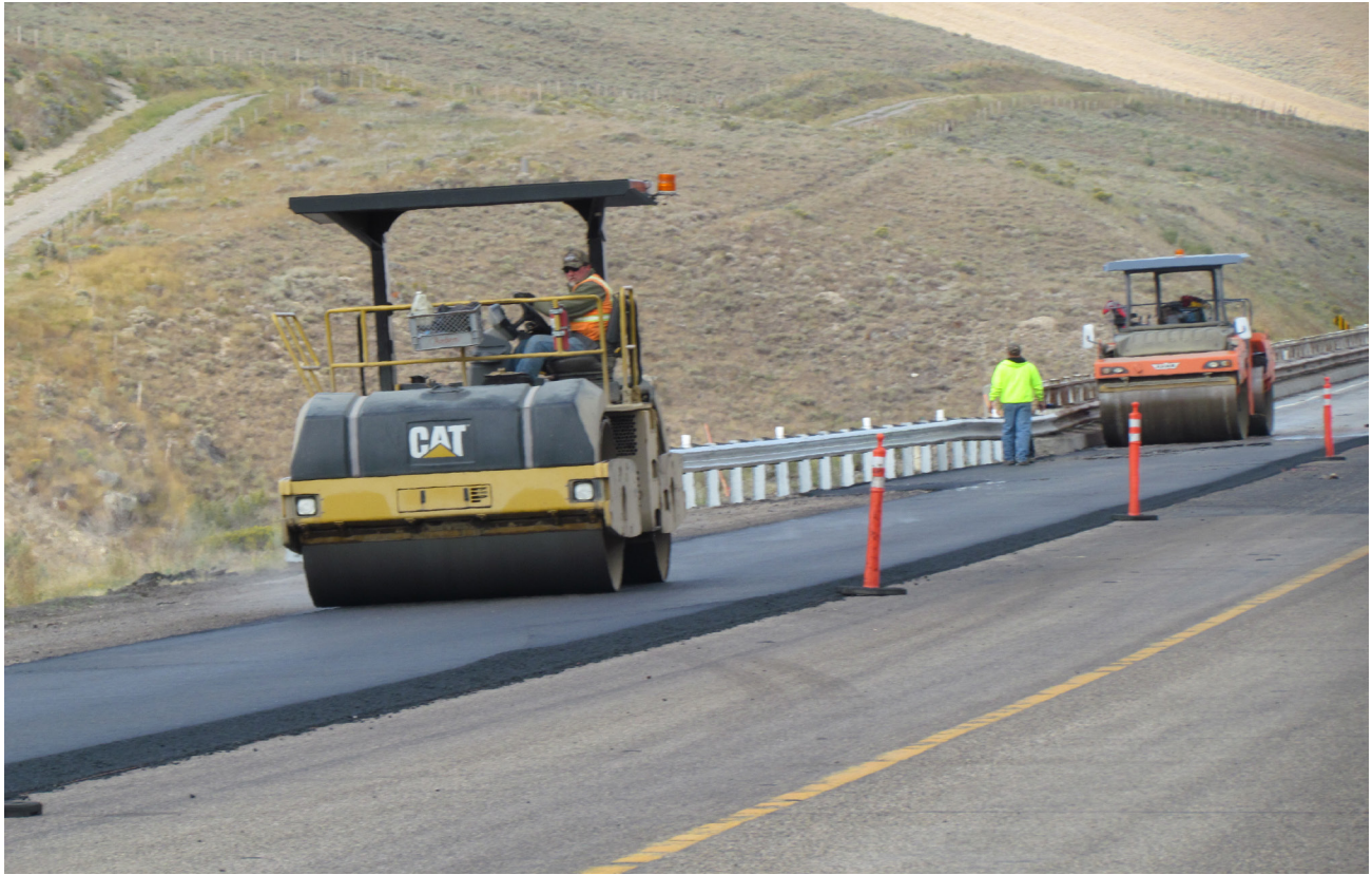
Figure 4- Beginning of Sasobit paving section, note the “wave” of plant mix in front of rollers
