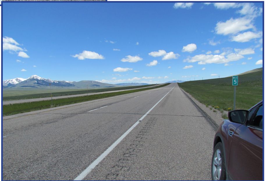
Figures 25 and 26- WMA treatment southbound (top) shows cracking near the centerline and missing seal and cover material and HMA northbound (right) exhibits similar conditions near RP 5
