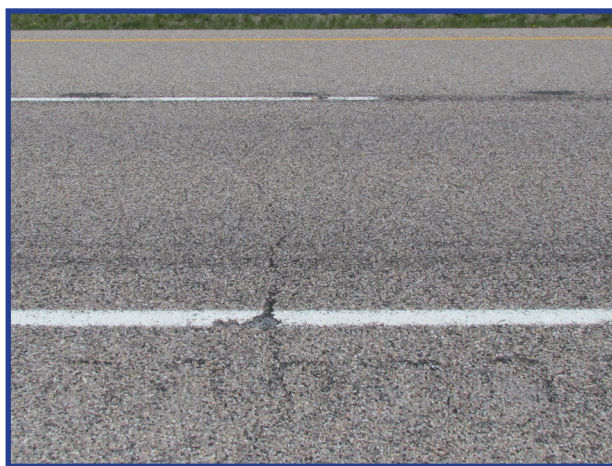
Figure 13- Examples of cover material loss along the roadway shoulder and center line in southbound lanes
