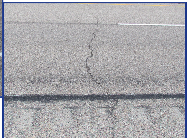
Figure 13- Examples of cover material loss along the roadway shoulder and center line in southbound lanes
