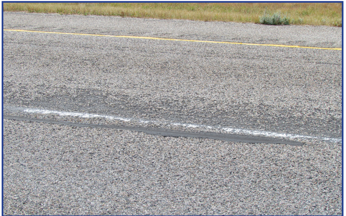
Figure 21- HMA northbound close-up shows cracking near the centerline and missing seal and cover material near RP 5
