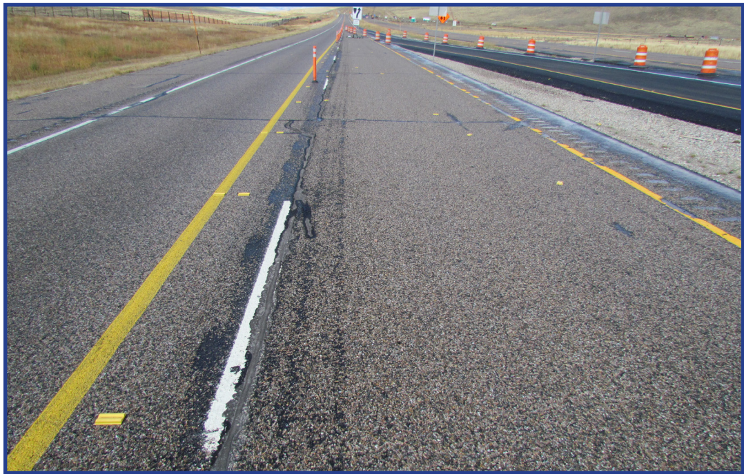
Figure 19- Foaming treatment southbound shows cracking near the centerline and missing seal and cover material near RP 1
