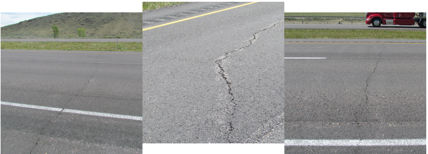
Figure 11- Examples of surface cracking in hot mix asphalt pavement in southbound lanes (left), warm mix asphalt pavement (center), and hot mix asphalt pavement in northbound lanes (right)
