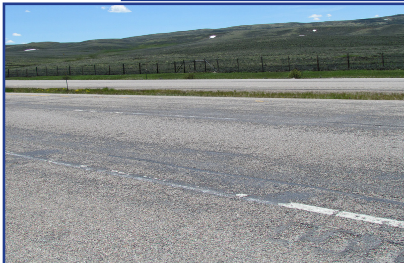
Figures 26- WMA treatment southbound shows missing seal and cover material near RP 1.5
