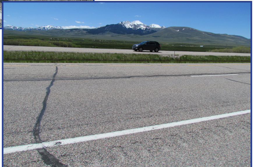
Figures 23 and 24- Evotherm treatment southbound (top) shows cracking near the centerline and missing seal and cover material and HMA northbound (right) shows the same conditions near RP 9
