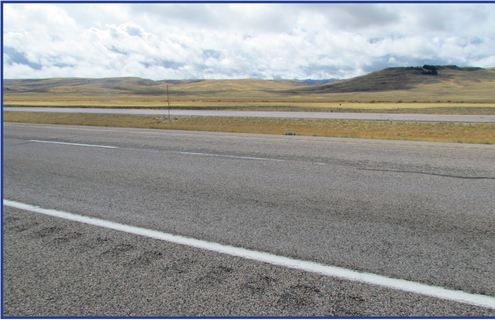
Figure 20- HMA northbound shows cracking near the centerline and missing seal and cover material near RP 5
