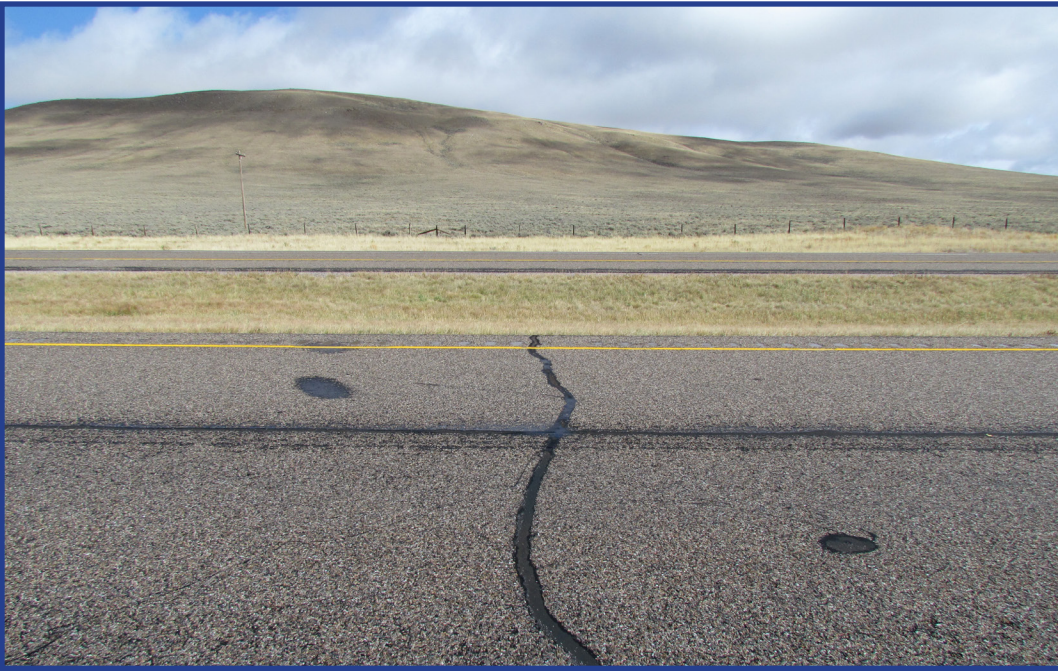
Figure 18- Reflective cracking and missing seal and cover material in southbound lane near RP 4.5
