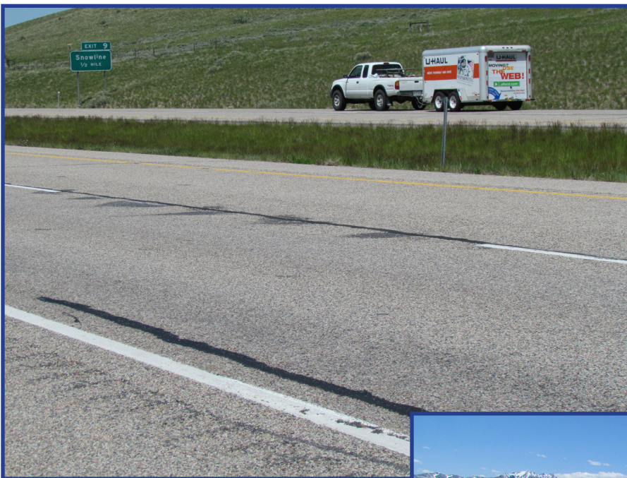
Figures 23 and 24- Evotherm treatment southbound (top) shows cracking near the centerline and missing seal and cover material and HMA northbound (right) shows the same conditions near RP 9
