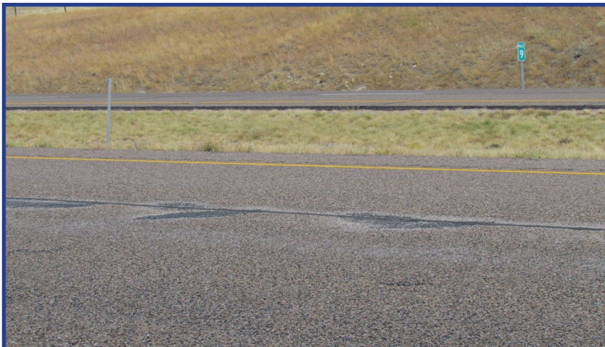
Figure 17- Evothrm treatment southbound shows cracking near the centerline and missing seal and cover material near RP 9
