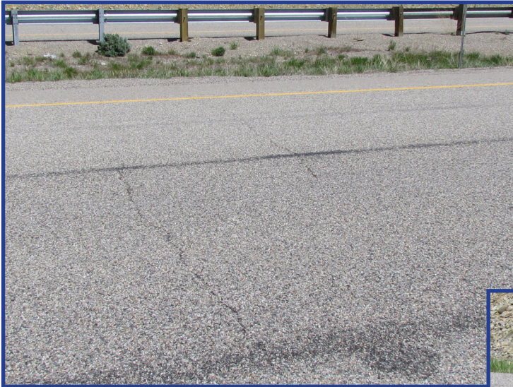
Figure 12- Examples of reflective cracking in warm mix asphalt pavement (top) and hot mix asphalt pavement in northbound lane (right)
