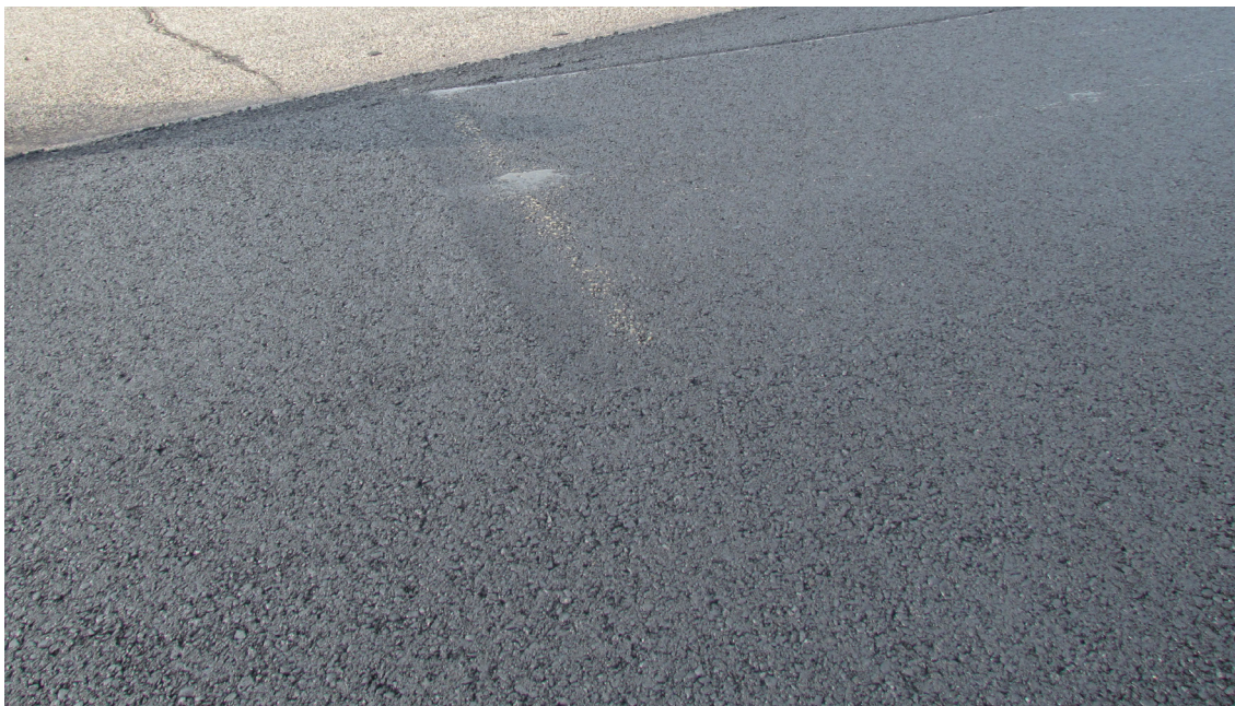
Figure 5- Beginning of Sasobit paving section when plant and placement temperatures were high
