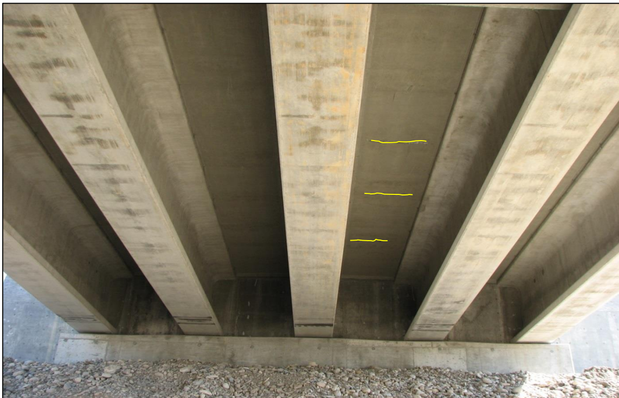
↑ East Bound Deck – East End: SRA/SPF placement .
