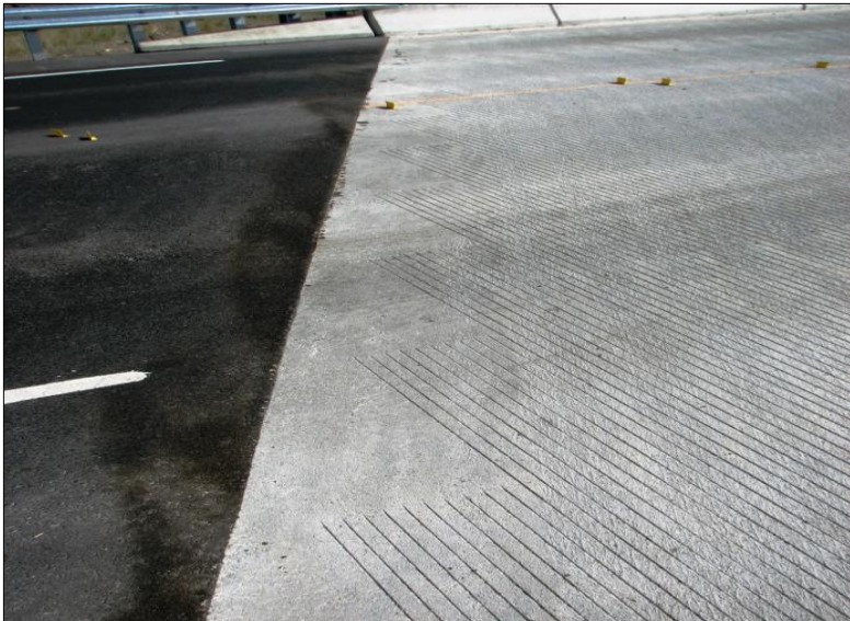
← Top side of west end of east bound deck; no visible cracking observed.
