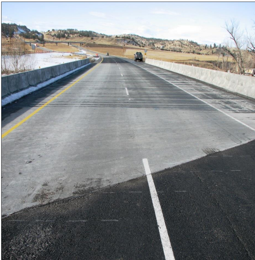
← Overview of deck; view west.
