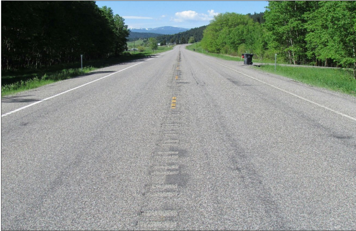
↑ Representative image of project centerline prior to permeant striping.
