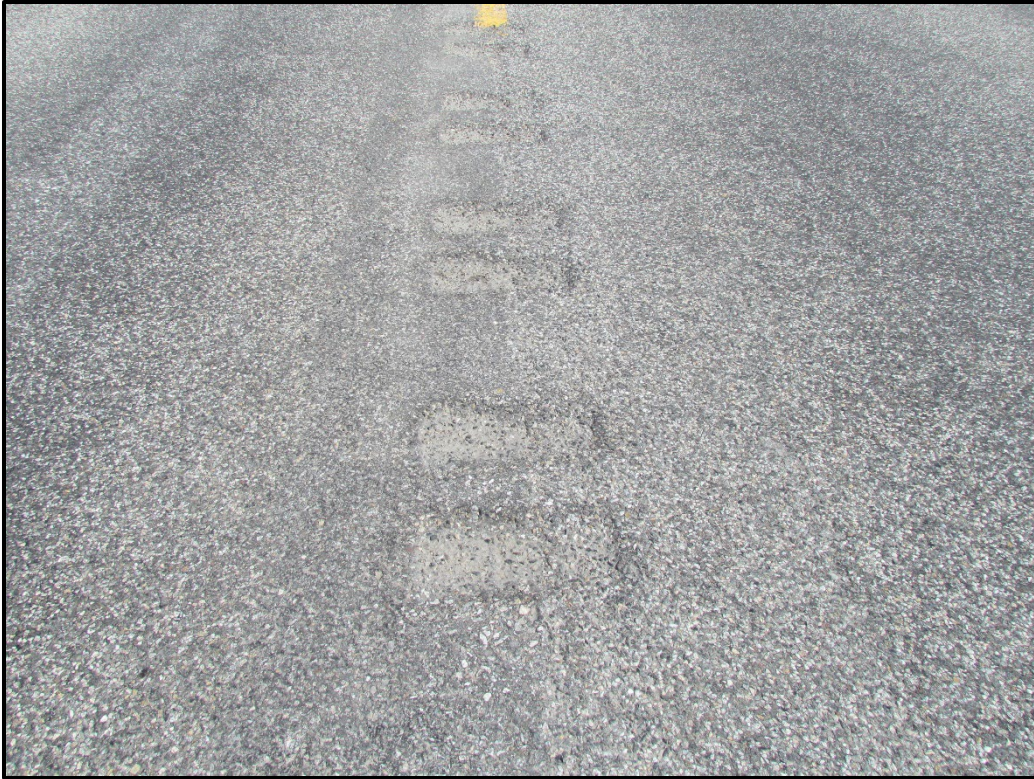
↑ Close-up of the centerline near RP 11.0.
