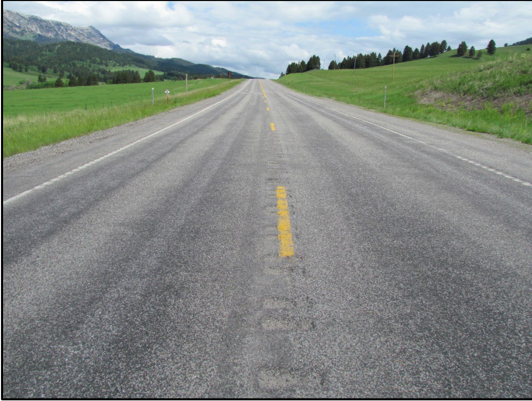
↑ RP 12.0, view north. No change in longitudinal joint condition.
