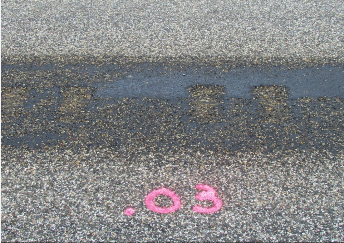
↑ Condition of Jointbond approximately 30 minutes after application.
