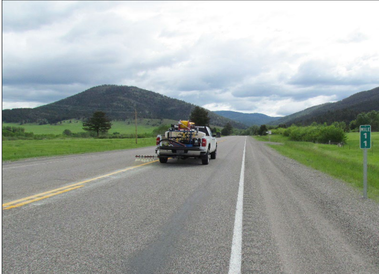
← Jointbond application starting at RP 11.0, view north.
