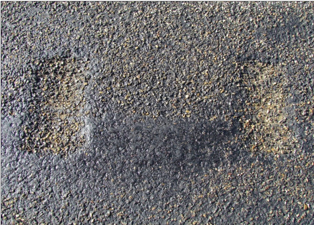
↑ Condition of Jointbond approximately 90 minutes after application.
