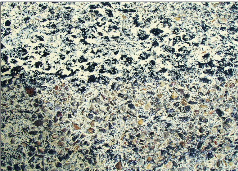
← Closer view of Jointbond after application.
