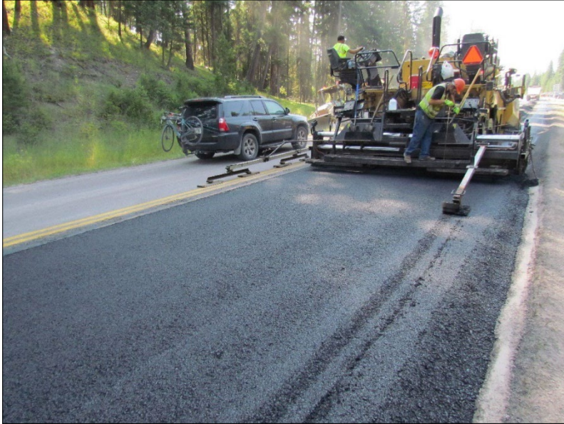
← Start of the southbound paving phase.
