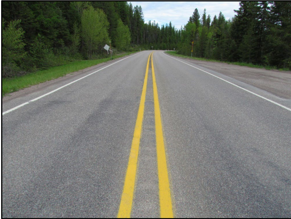
↑ RP 31.5, view north. Conditions at the south end of the project.
