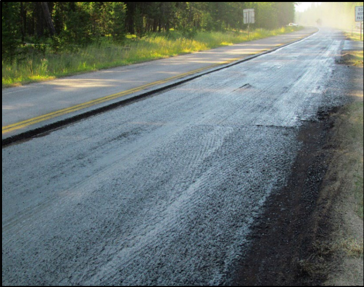
← Completed tack run.
