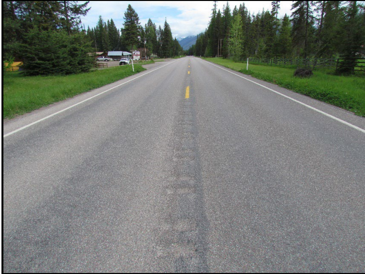
← RP 38.3, view north. Area where the VRAM bleed through is a little more noticeable.
