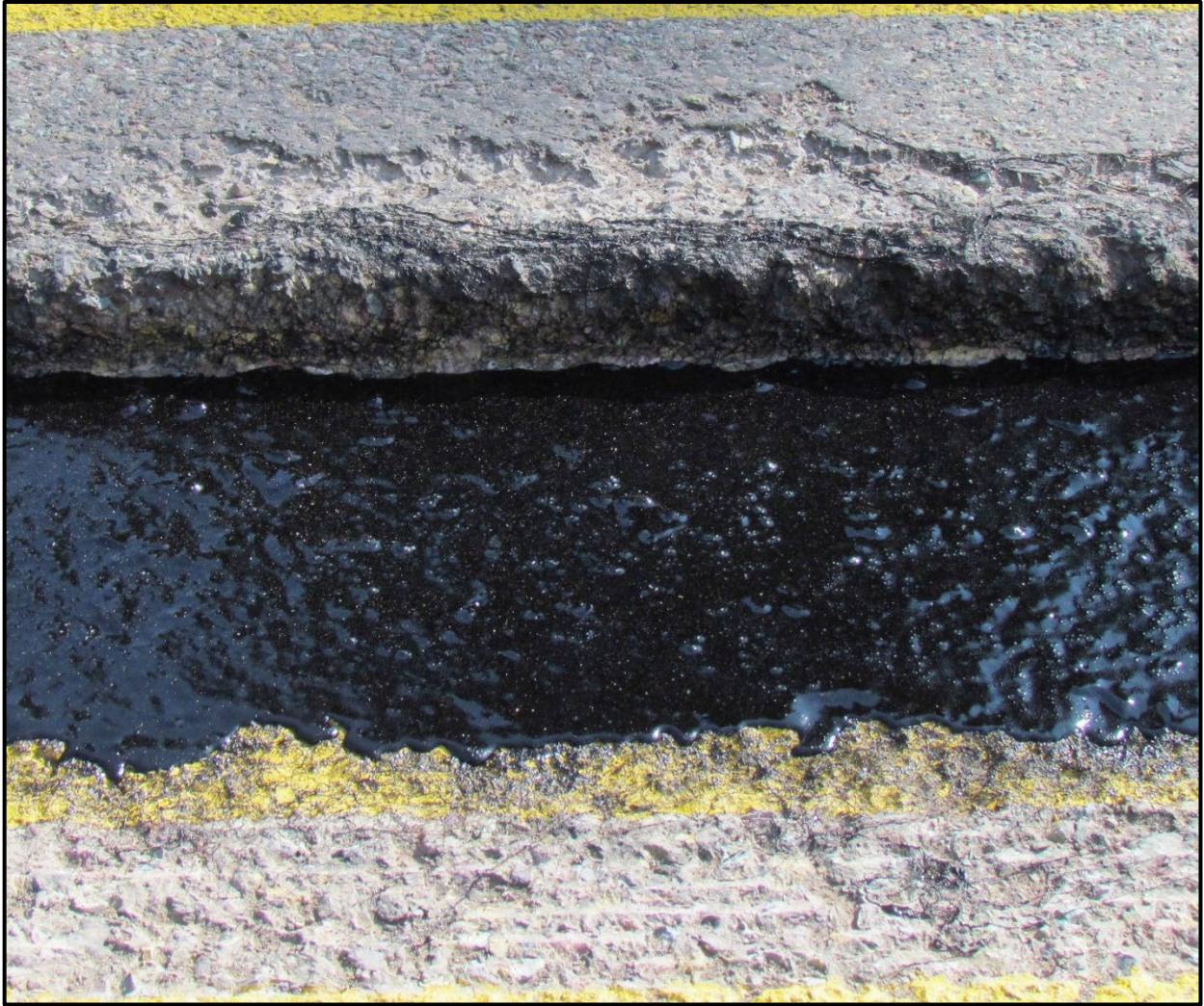
↑ Close-up of VRAM with an approximate cure of 15 minutes (southbound lane).
