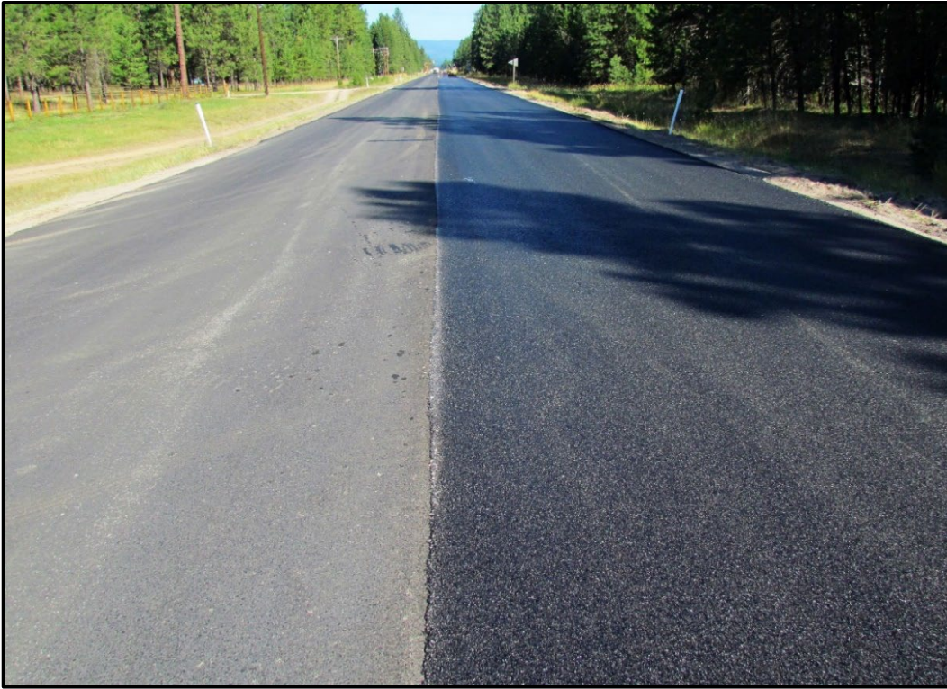
↑ Northbound lane paving completed.
