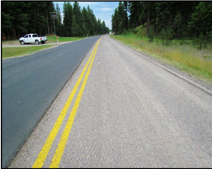
← Northbound lane milled and prepped for VRAM application.
