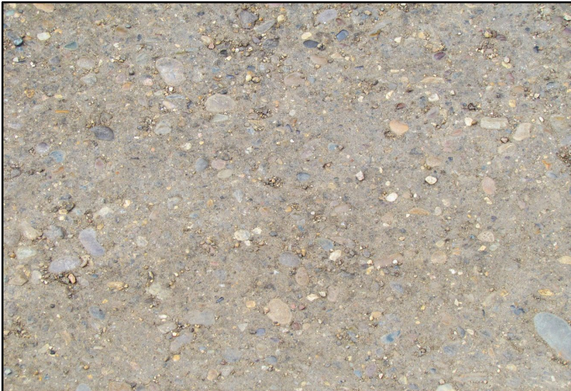
↓ Close-up of compacted base.
