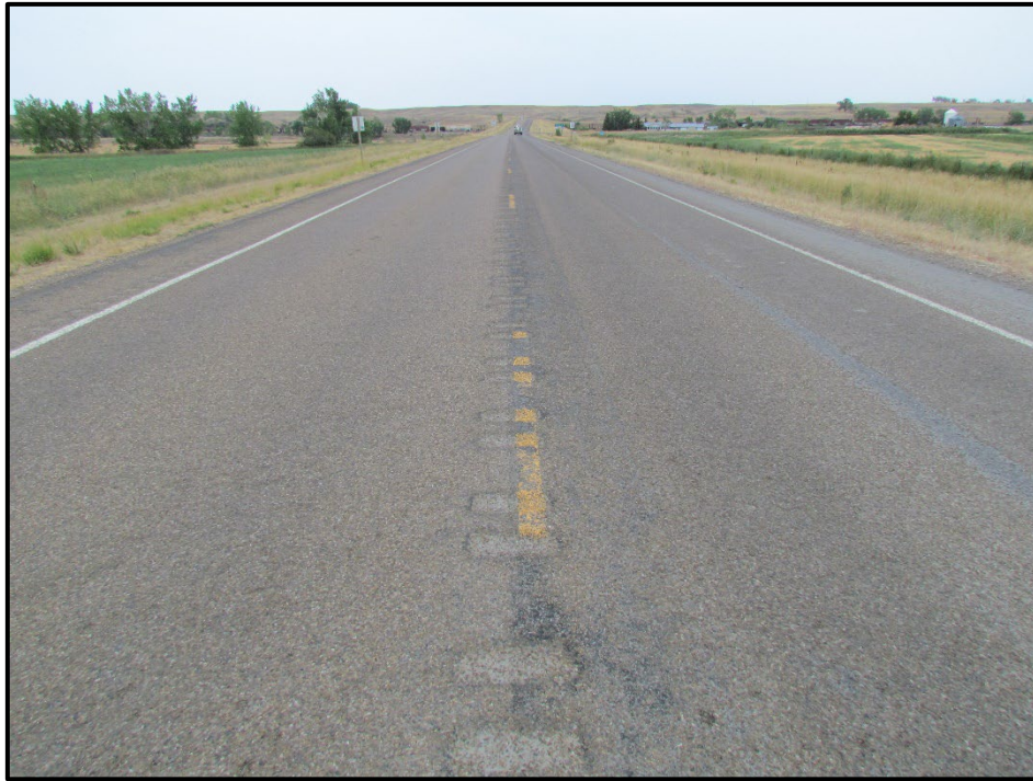
↑ Example of pavement conditions in section 1, view north.
