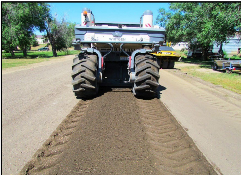
← Rear view of the Wirtgen unit and blended base.
