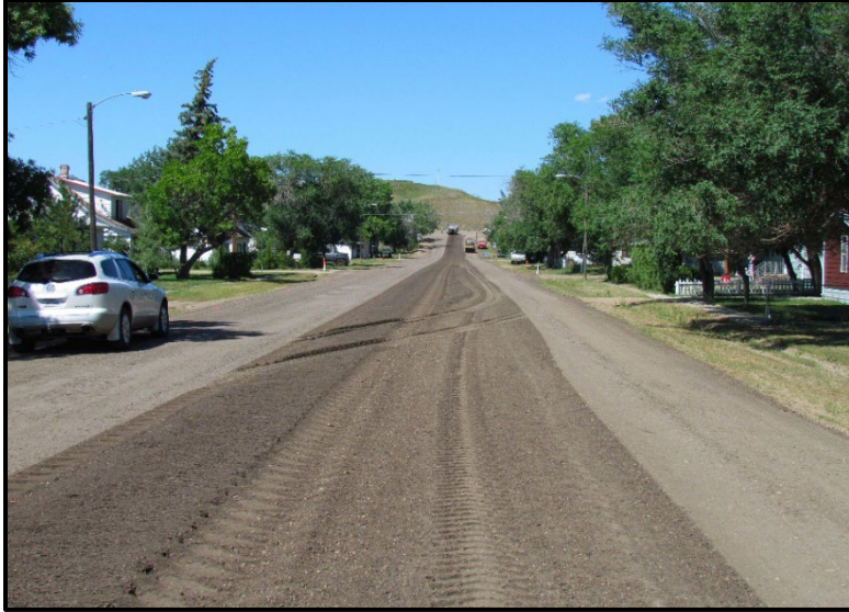
← Completed pass, Sargent St. view north. Prior to compaction.
