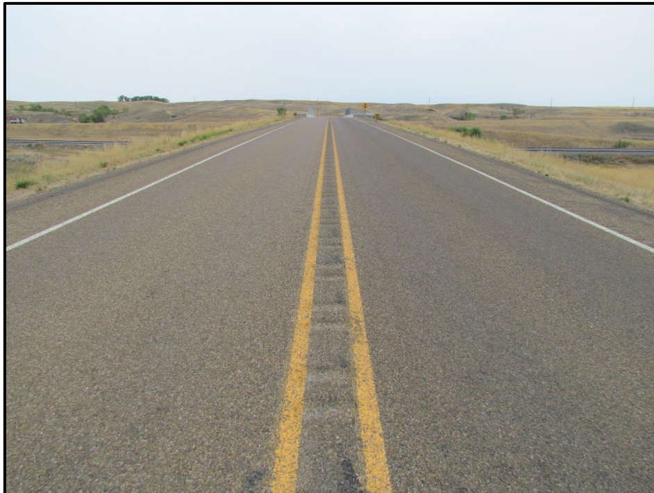
↑ Example of pavement conditions in section 2, view north.
