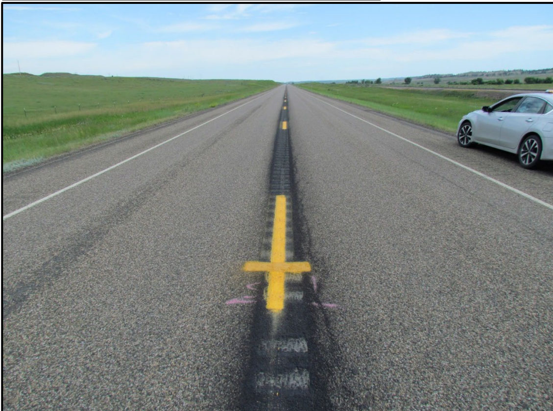
↓ The SCLRS was fog sealed (SS-1) and restriped, view north.
