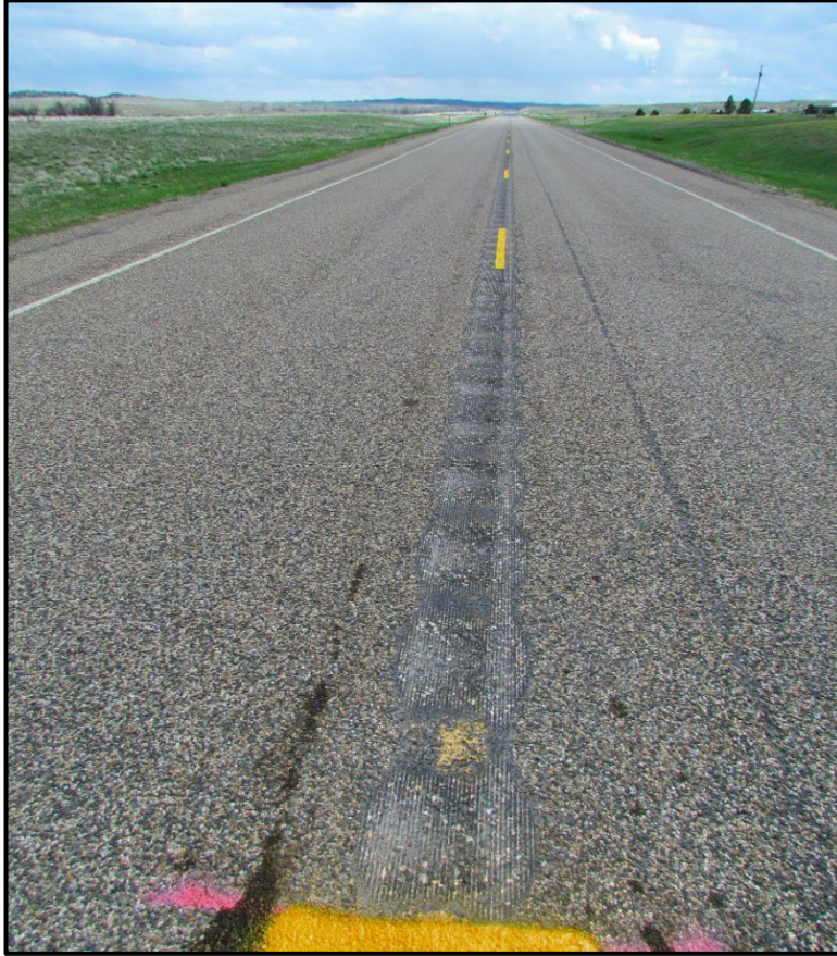
← Additional image of SCLRS mill with temporary striping, view north.
