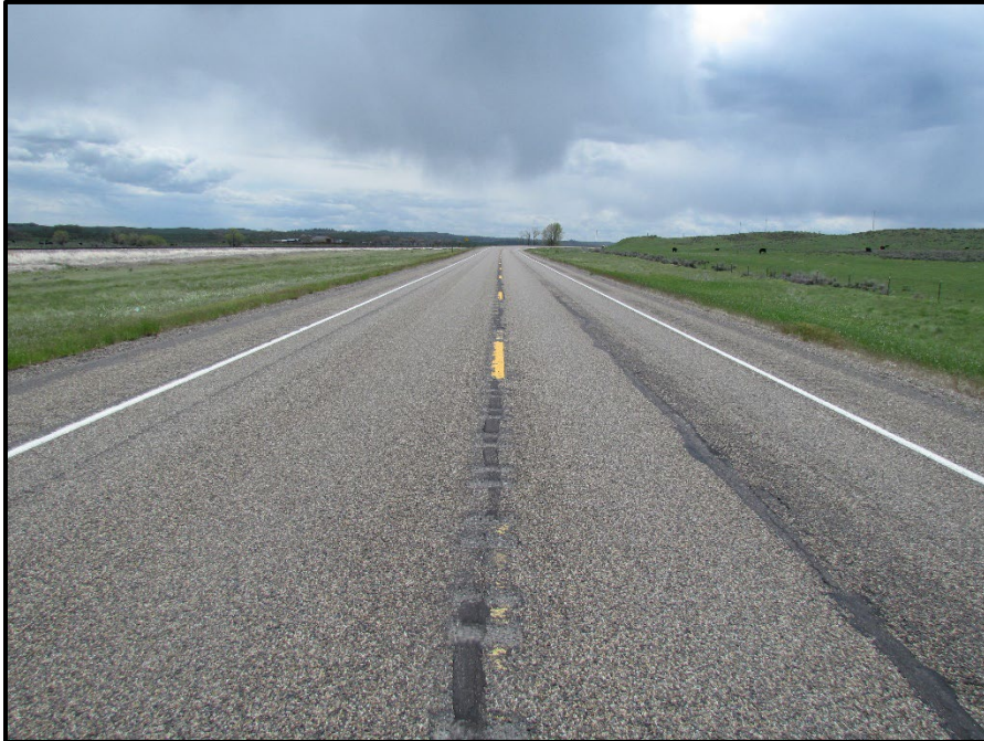
← Control section of standard center line rumble strips just south of test section 1 near RP 31.0.
