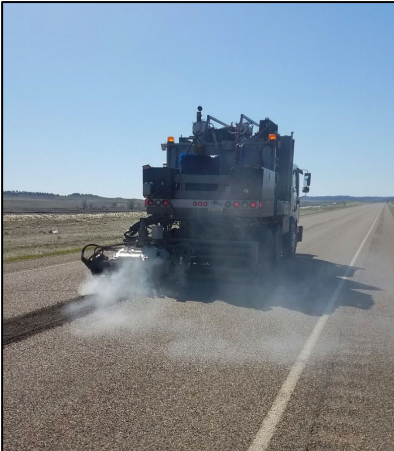
◀ Rear view of the SPT Noiseprint Rumble Strip Mill truck in operation.
