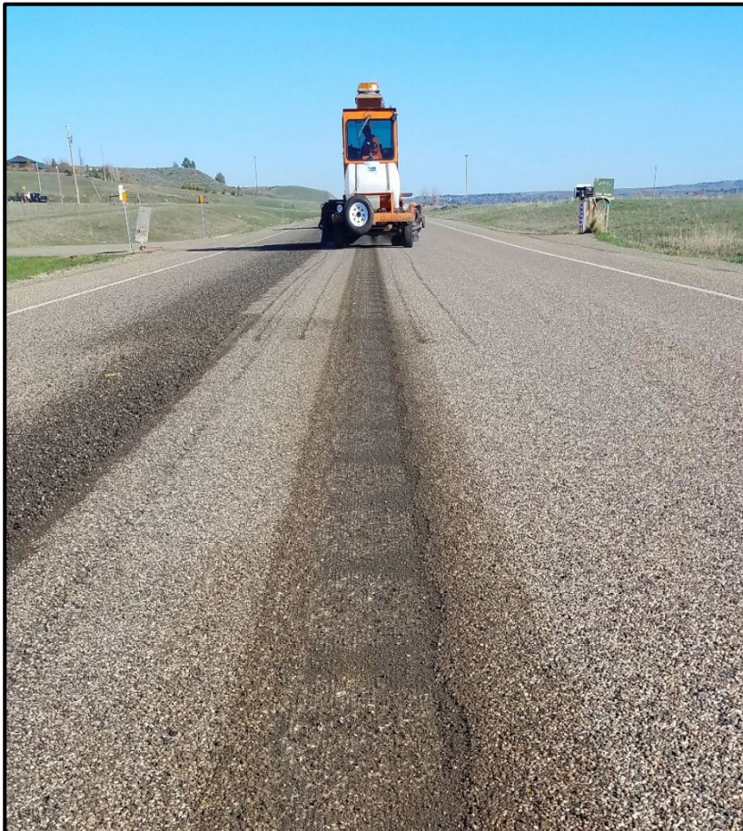
← Sweeper performing the SCLRS clean-up prior to the application of the temporary striping.
