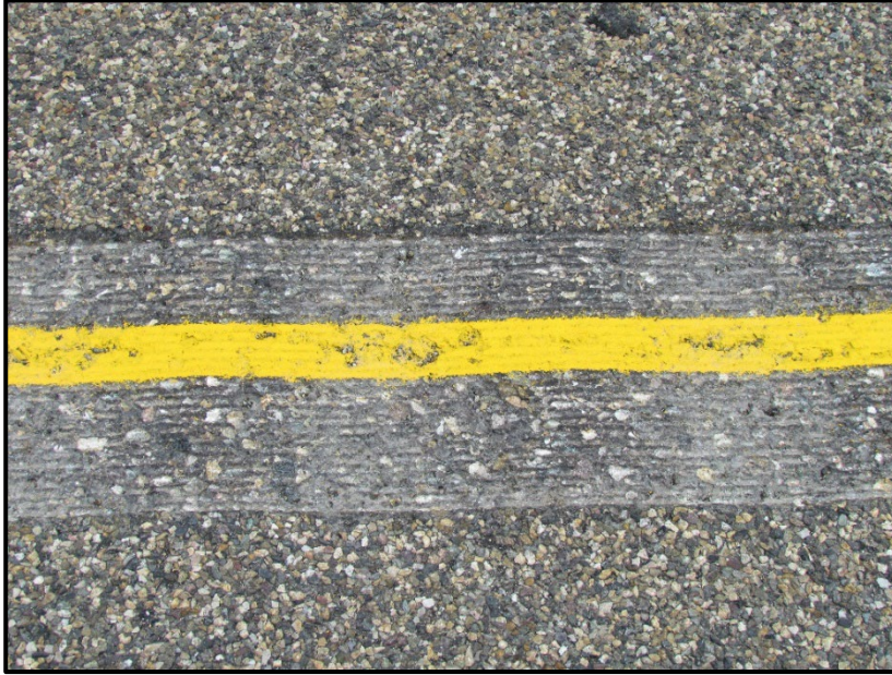
↙↓ Close-up of SCLRS cut with temporary striping. Lower image is overview of rumble strip section, view north.
