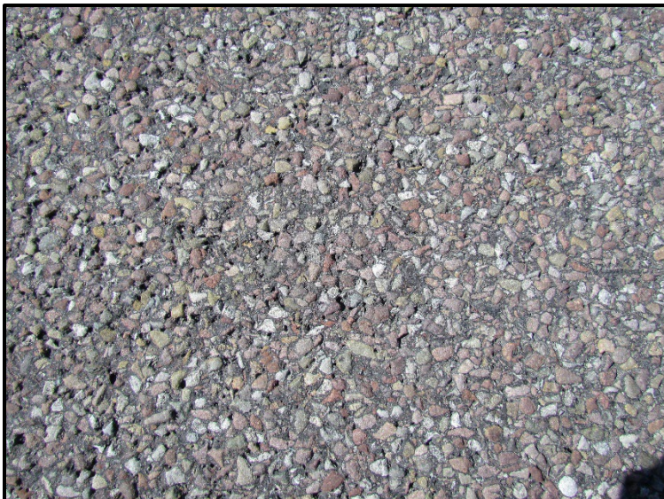
← Close up view of an example of the 3/8" PMS texture.
