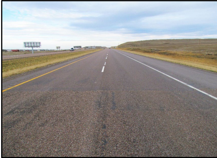
← RP 283, view north, transition from \frac{3}{4} " PMS with chip seal (control) to \frac{3}{8} " PMS without chip seal (test).
