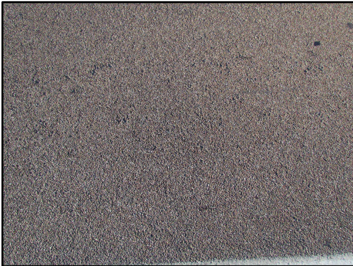
← ↓ View of 3/4" PMS with chip seal surface texture at varying distances.
