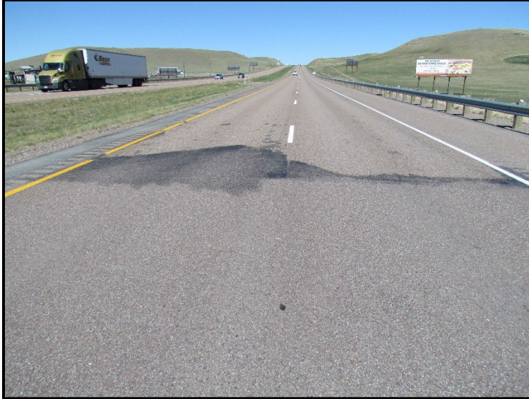
← RP 284, view north. Transition from 3/8" PMS to 3/4" PMS with chip seal.
