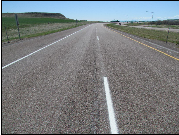
← RP 283, view south. View of the chip seal on 3/4" PMS.
