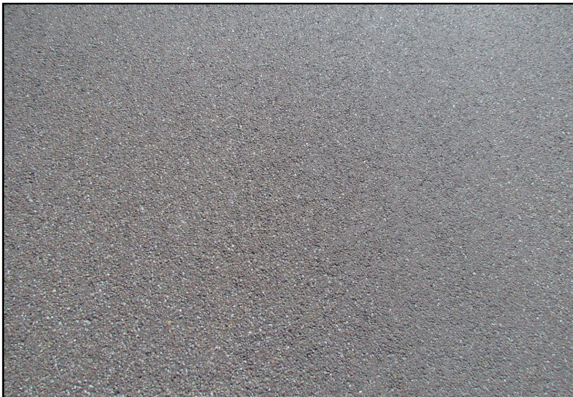
↑ RP 283, view north, transition point of control to test section. ↓ Representative image of the 3/8" PMS texture.
