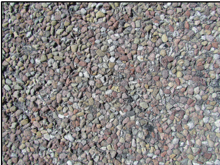
← Close up view of an example of the chip seal texture.
