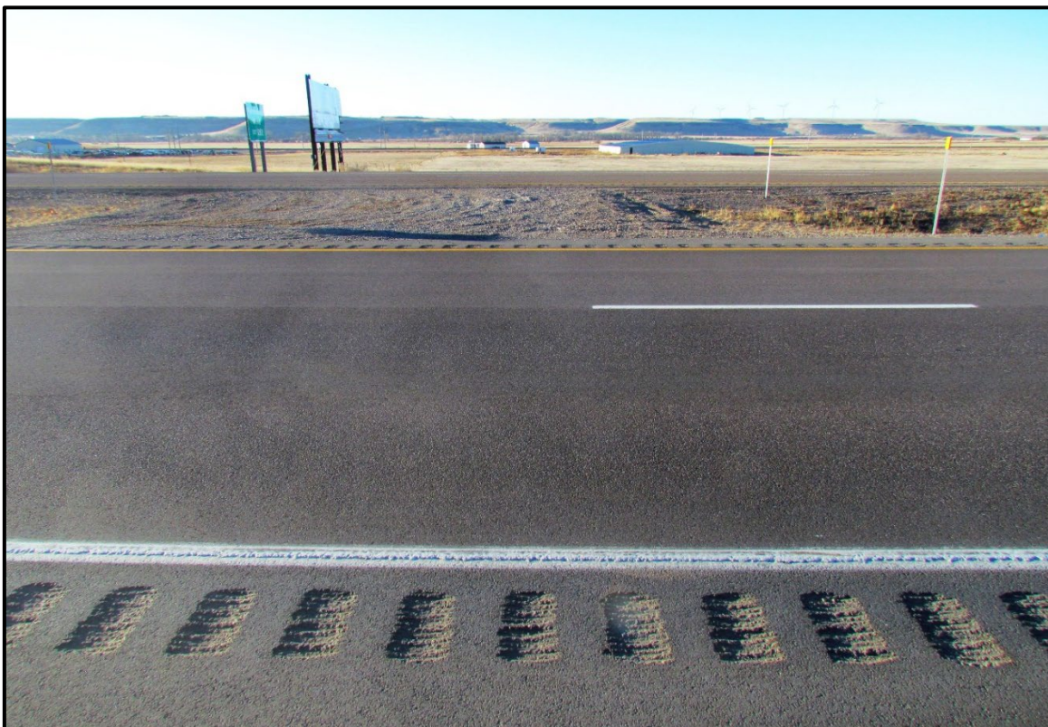
↕↔ Representative images of the 3/8" PMS at approximate RP 283.5. Above is view north.
