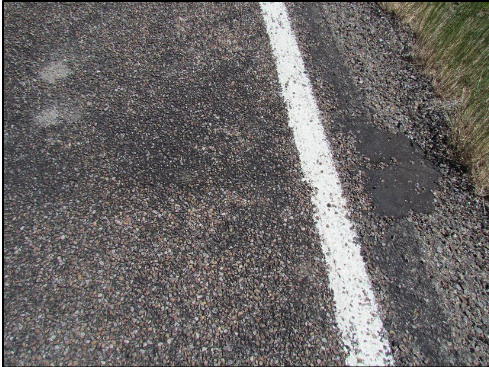
↑ Close up view of Mastic One. The mastic is bleeding through the chips, but the chips are holding for the majority of the mastic sections.
