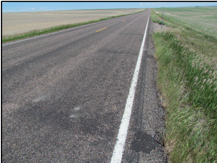
← RP 14, view of some Mastic One showing through the chip seal.
