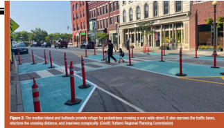
Figure 2: The median island and bollards provide refuge for pedestrians crossing a very wide street. It also narrows the traffic lanes, reduces the crossing distance, and improves visibility. Credit: Rutland Regional Planning Commission
