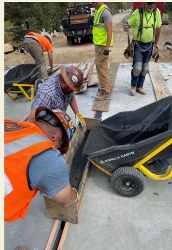
MT-UHPC being placed into keyways.
