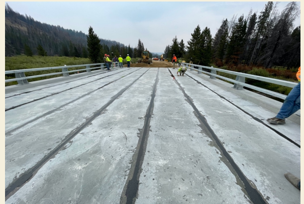
Bridge with epoxied MT-UHPC keyways.
