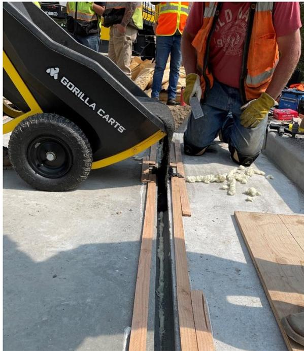
Figure 4: UHPC directly added to keyway with 1/2-in strip for overcasting
