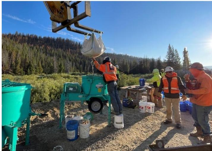
Figure 2: Sack of dry mix being added to the mixer
