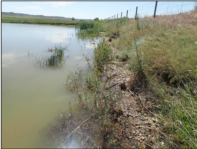
Additional Photo 1: bank erosion along S fence line Year: 2024
