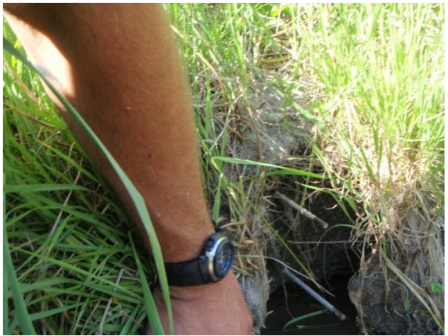
Bank Erosion Pin #1 Taken in 2011
