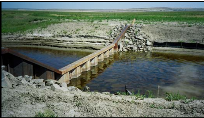
Photo 5: Sheet Pile Diversion Structure.
