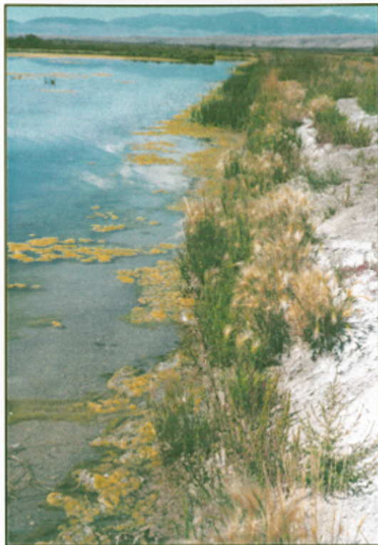
Photo Point 7: Eroding dike east of photo point 7.
