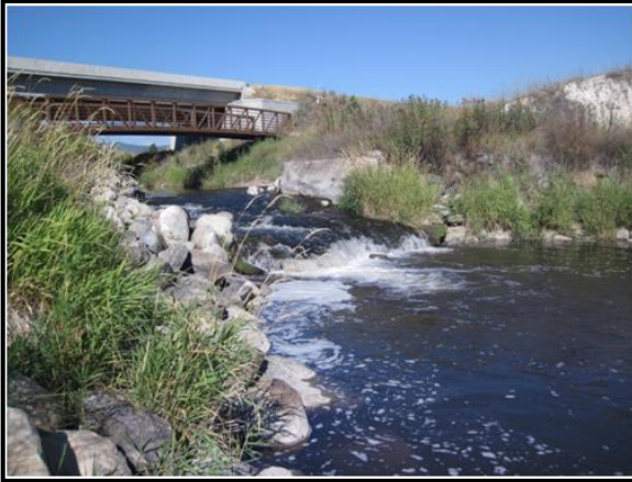
Photo Point 1: View of grade control structure downstream of project area. Compass: 315° (Northwest)
