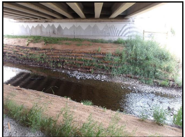
Additional Photo 3: Upstream end of eroding south bank under the US 93-Kalispell Bypass bridge.
