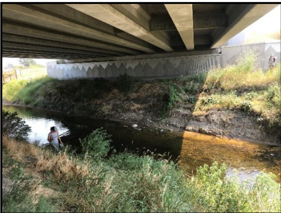
Additional Photo 3: Upstream end of eroding south bank under the US 93-Kalispell Bypass bridge.
