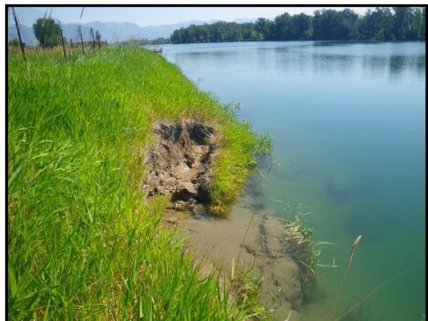
Additional Photo 2: Bank calving off behind coir soil lift at Transect 4.
