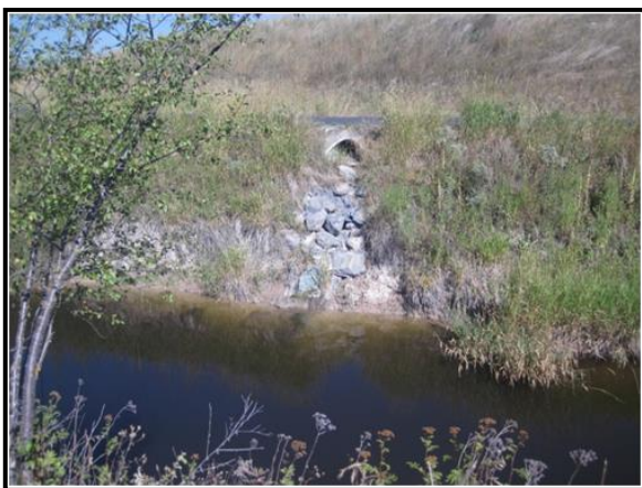
Additional Photo 6: Stabilized culvert outlet.
