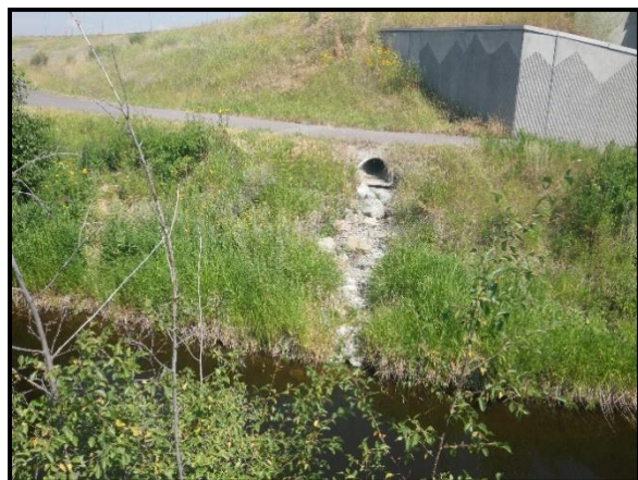
Additional Photo 6: Stabilized culvert outlet.
