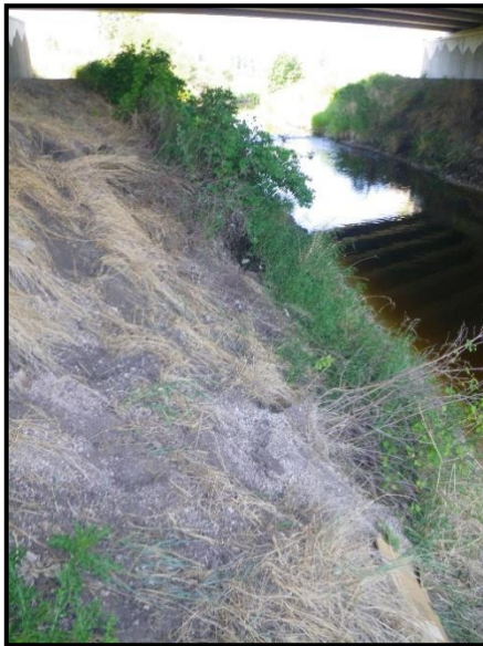
Additional Photo 8: Toe of eroding bank EBR1-2 showing bank sloughing and loss of woody vegetation.
