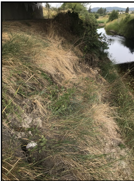
Additional Photo 8: Toe of eroding bank EBR1-2 showing bank sloughing.
