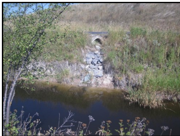
Additional Photo 6: Stabilized culvert outlet.
