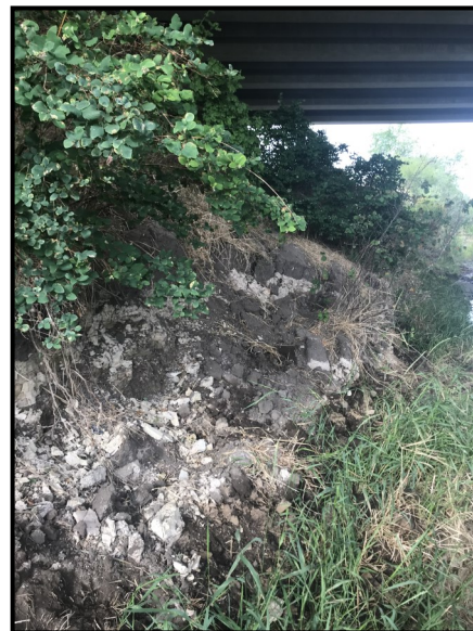
Additional Photo 9: Toe of eroding bank EBR1-2 showing loss of woody vegetation.
