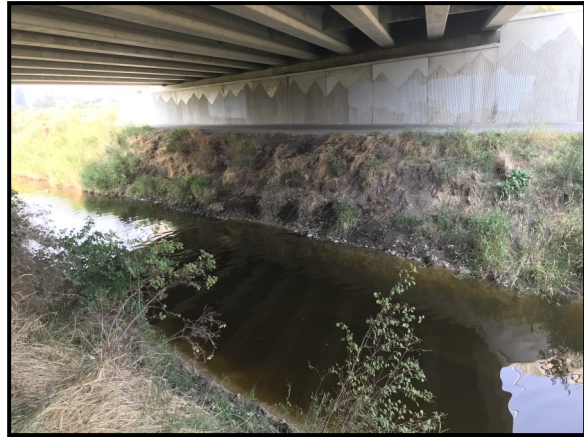
Additional Photo 7: Eroding Bank EBL2
