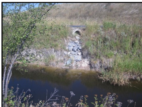
Additional Photo 6: Stabilized culvert outlet.
