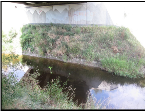
Additional Photo 7: Eroding Bank EBL2
