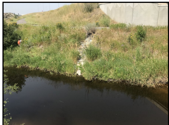
Additional Photo 6: Stabilized culvert outlet.
