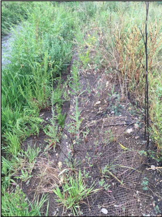
Additional Photo 5 Description: Unvegetated upper soil lift Taken in 2016 @ STA 11+00
