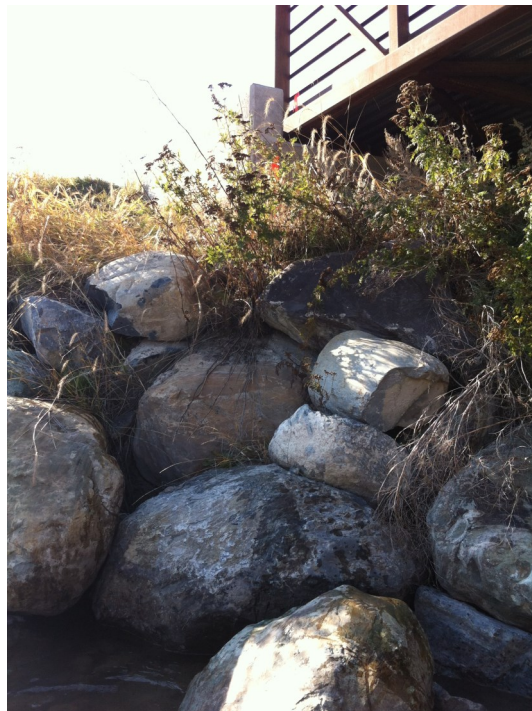
Transect 4 Right Looking South Riprap D-17
