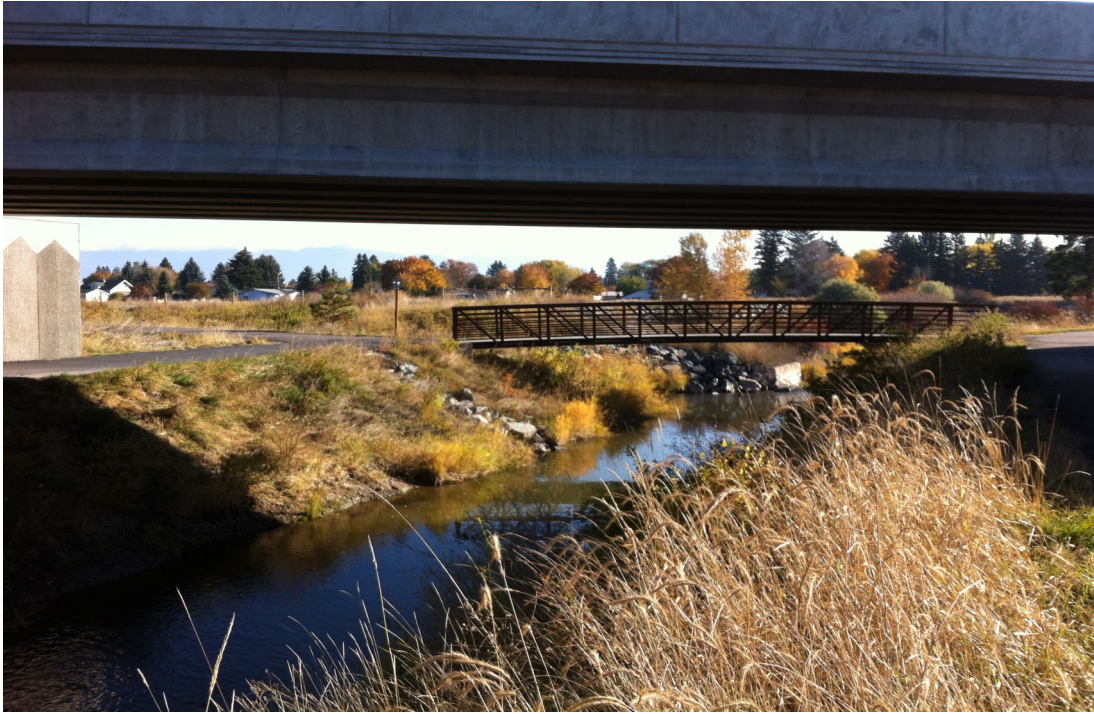
West of Bridge Looking Downstream East
