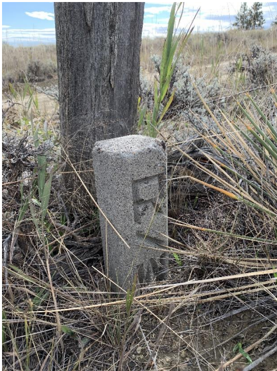
Figure 6-3: Concrete right-of-way marker
