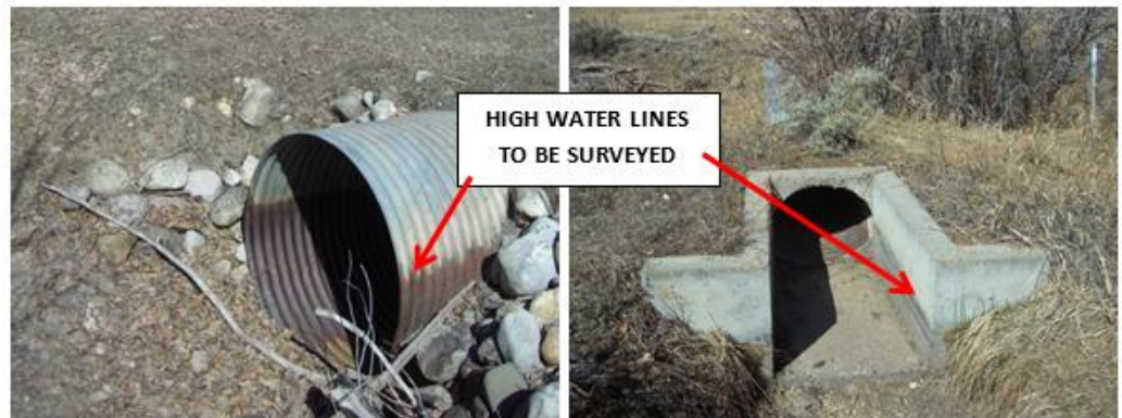
Figure 5-8: Irrigation highwater marks
