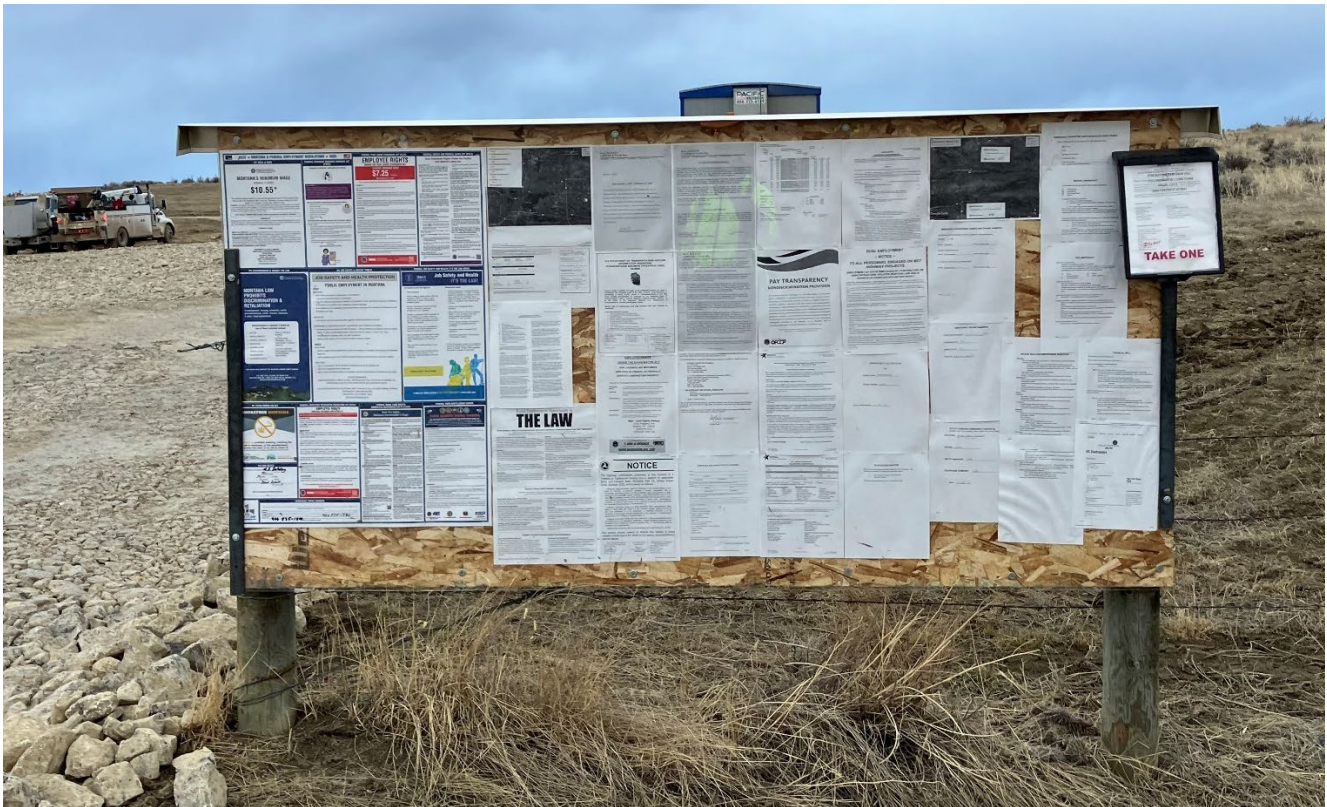
Required notices and posters are posted on particle board which is mounted on posts. Contract-specific items are in the outdoor brochure holder in the top right corner.
