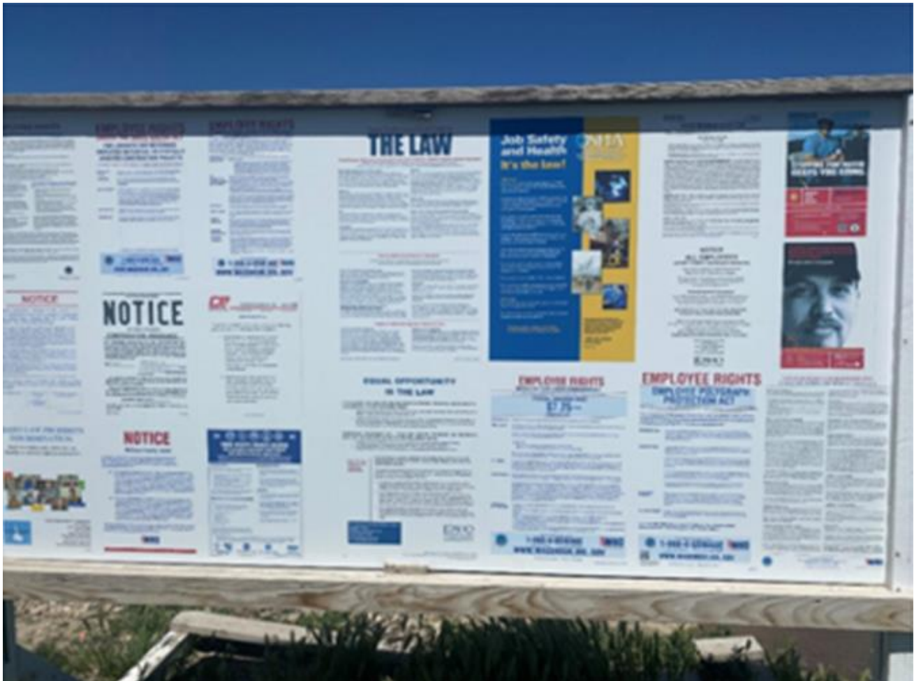
Required notices and posters are printed on MDO which is framed and mounted on posts.
