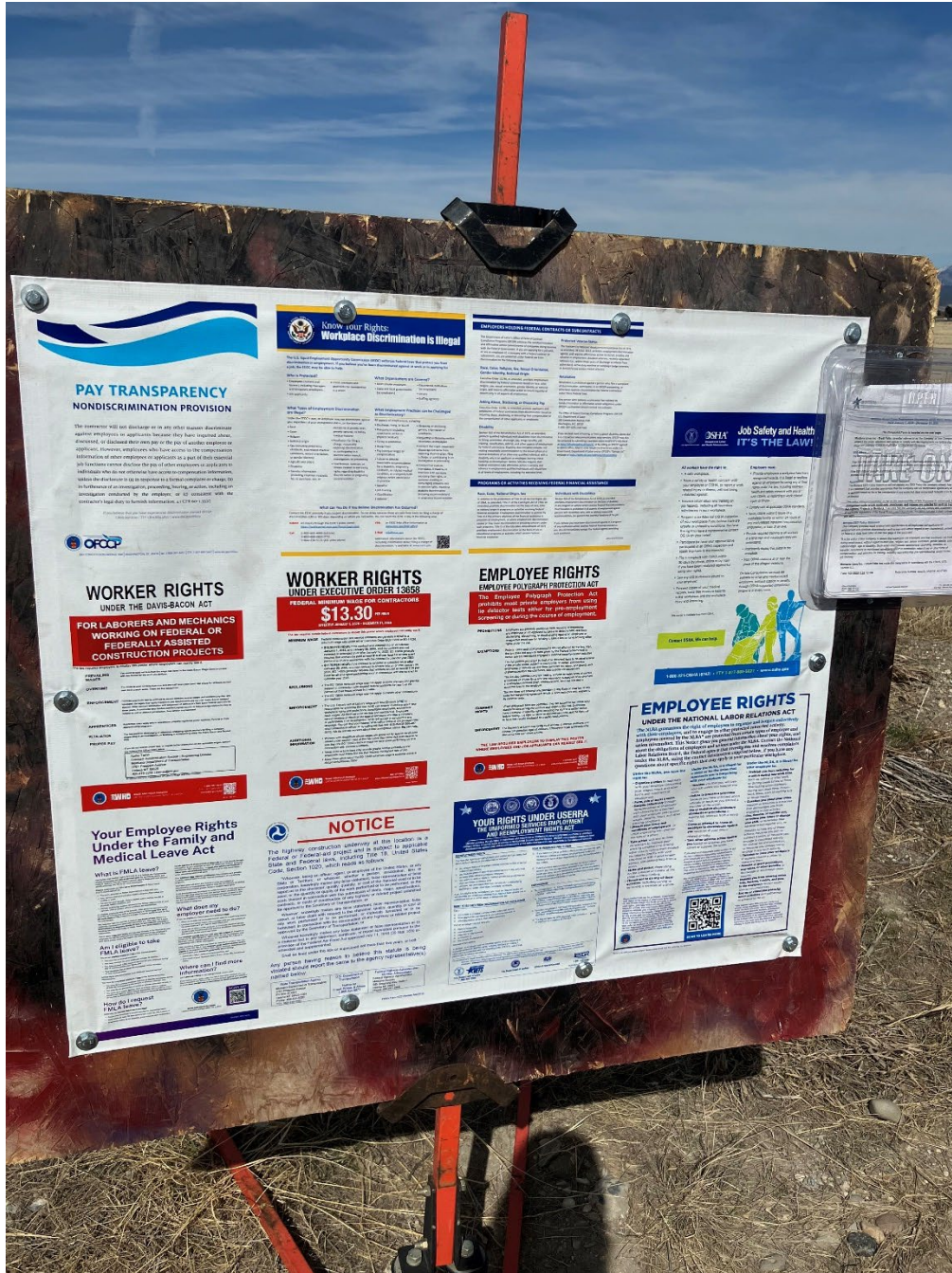
Required notices and posters are on banner material, fastened to a piece of plywood, and held by a wind jammer. Wage rates and EEO Policy Statements are in the outdoor brochure holder (top right corner).
