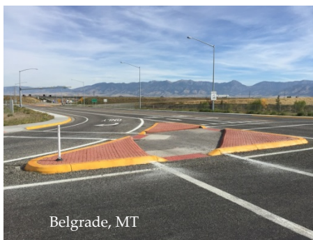
Exhibit 7-20 Crossing Island with Channelization
