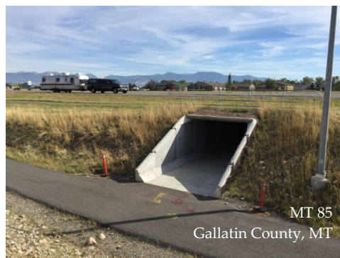
Exhibit 7-25 Grade Separated Crossing - Underpass
