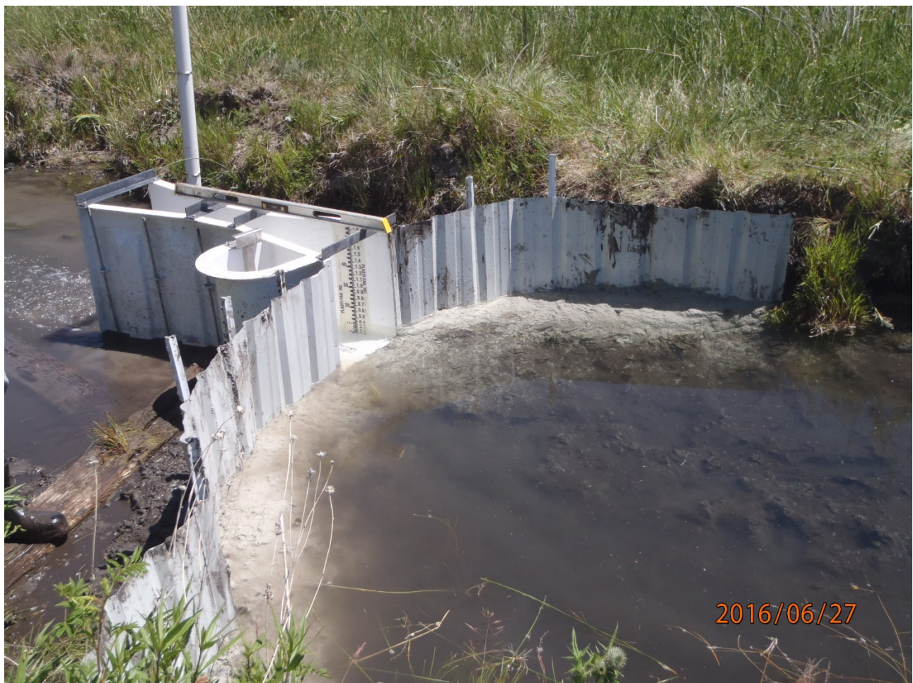
Photograph 1. Original Installation of 6-inch Parshall Flume
