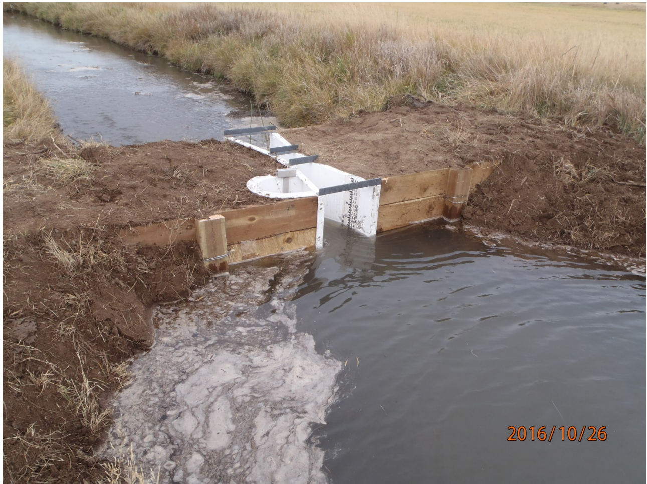
Photograph 2. Re-installation of 6-inch Parshall Flume by R.E. Miller and Sons
