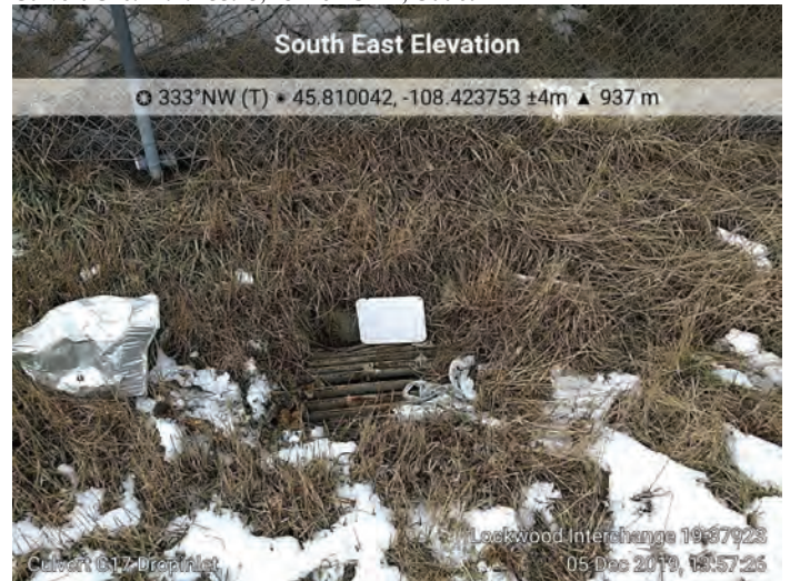
Culvert C17. M.P. 454.73, 24-inch RCP, Drop Inlet
