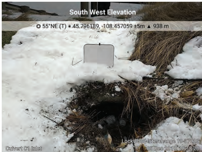
Culvert C1. M.P. 452.84, 24-inch RCP, Inlet
