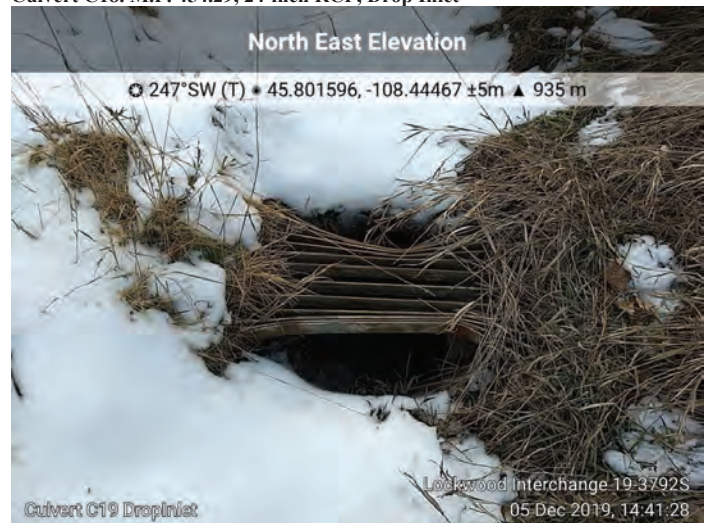
Culvert C19. M.P. 453.55, 24-inch RCP, Drop Inlet
