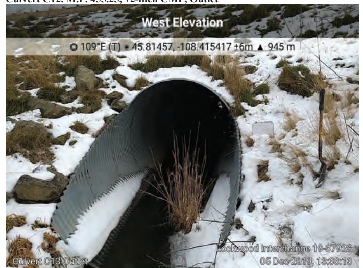
Culvert C13. M.P. 455.25, 90-inch CMP, Outlet
