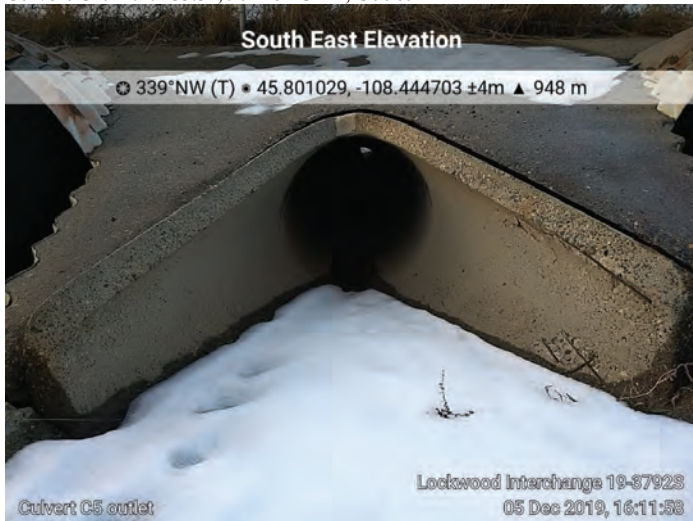
Culvert C5. M.P. 453.54, 24-inch RCP, Outlet
