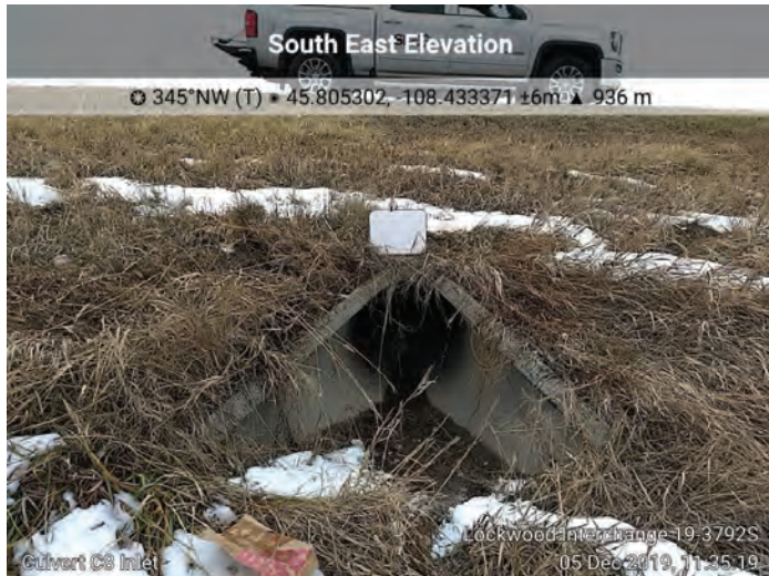
Culvert C8. M.P. 454.15, 24-inch RCP, Inlet
