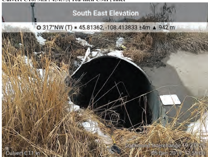
Culvert C11. M.P. 455.27, 72-inch CMP, Inlet
