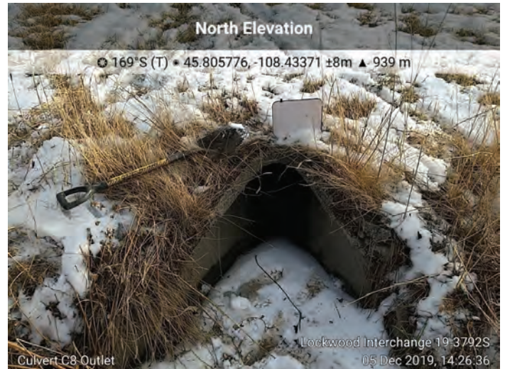
Culvert C8. M.P. 454.15, 24-inch RCP, Outlet
