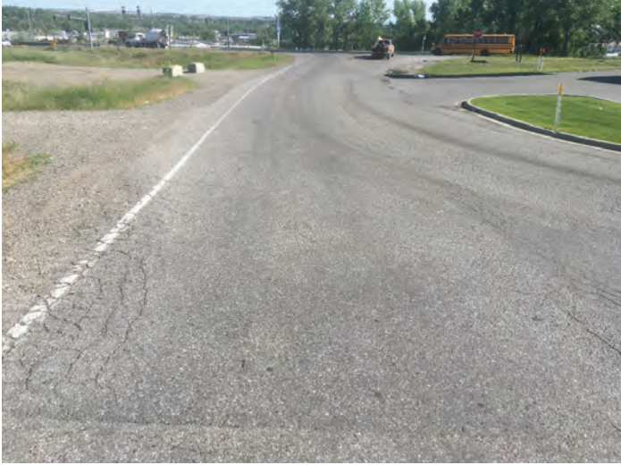
Coburn Road approach to Highway 87, looking northeast. Alligator and block cracking. Many shoulder failures.
