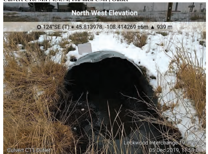
Culvert C11. M.P. 455.25, 72-inch CMP, Outlet
