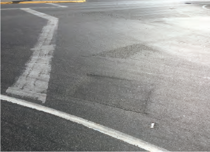
Highway 87 turn to I-90 westbound on ramp. A recent mill and overlay was performed, and bleeding was observed.
