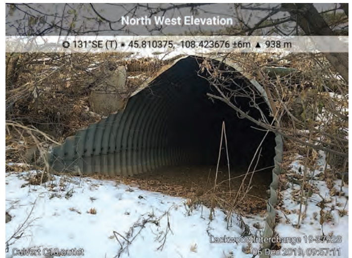
Culvert C10. M.P. 454.74, 102-inch CMP, Outlet
