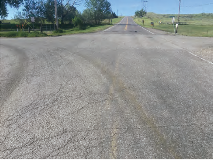
Coburn Road approach to Highway 87, looking southwest. Alligator and block cracking. Many shoulder failures.
