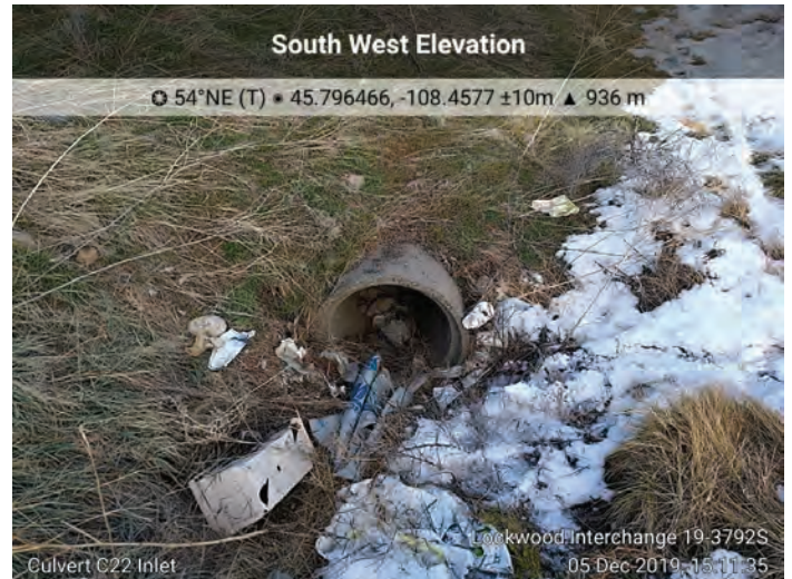
Culvert C22. M.P. 452.83, 24-inch RCP, Inlet
