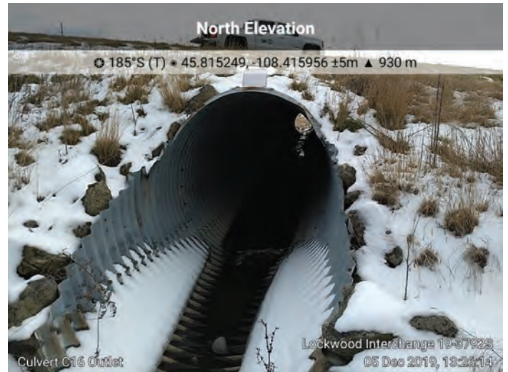
Culvert C16. M.P. 455.25, 78-inch CMP, Outlet
