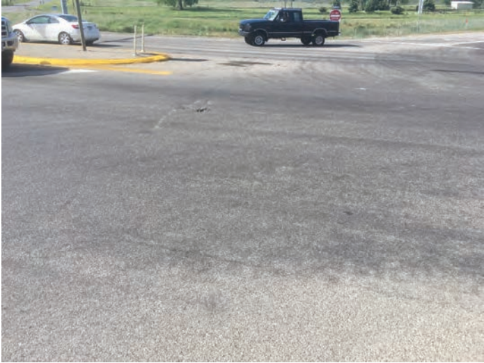
Highway 87 Lockwood Interchange south bridge end pavement distress, looking west. Pothole in intersection, and transverse crack. Intersection in poor shape beneath surface.
