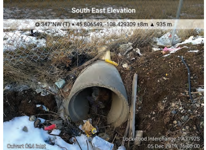
Culvert C24. M.P. 454.39, 24-inch RCP, Inlet
