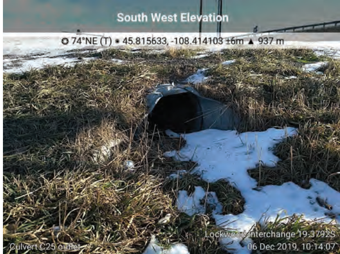
Culvert C25. M.P. 455.39, 24-inch CMP, Outlet
