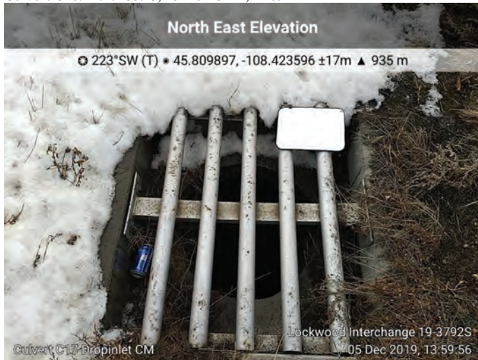
Culvert C17. M.P. 454.73, 24-inch RCP, Drop Inlet
