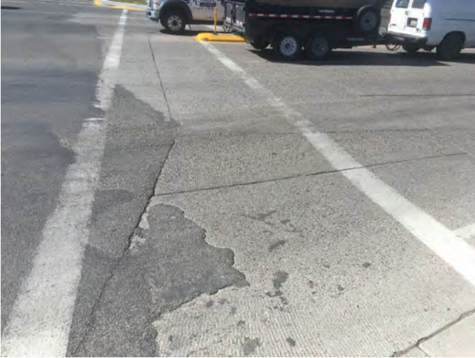
Intersection of Highway 87 and North Frontage Road, looking southwest. Closeup of drainage concern in low lying PCCP lane, with asphalt patches.
