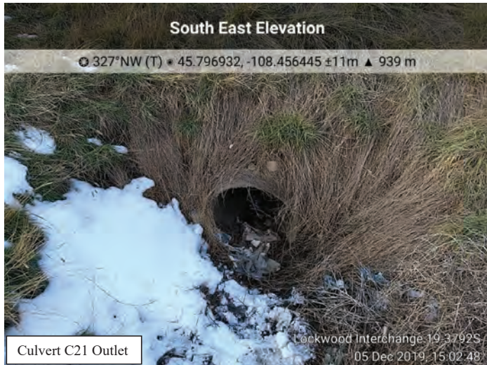
Culvert C21. M.P. 452.91, 24-inch RCP, Outlet
