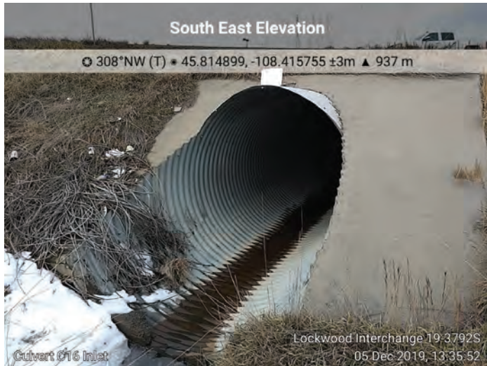
Culvert C16. M.P. 455.25, 78-inch CMP, Inlet
