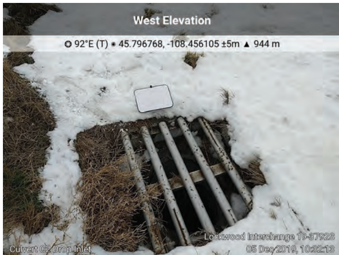
Culvert C2. M.P. 452.90, 24-inch RCP, Drop Inlet
