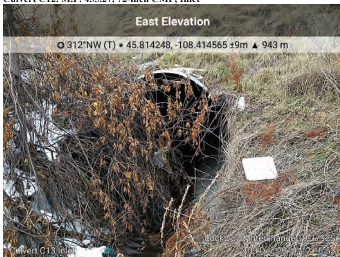
Culvert C13. M.P. 455.26, 90-inch CMP, Inlet
