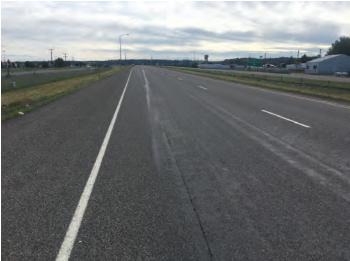
I-90 eastbound and westbound mainline, typical longitudinal crack.
