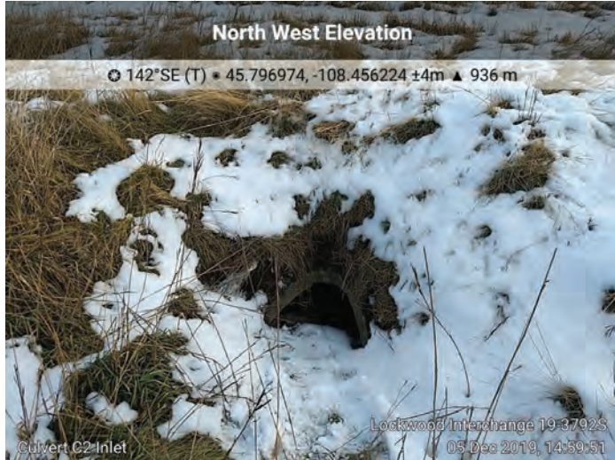
Culvert C2. M.P. 452.91, 24-inch RCP, Inlet
