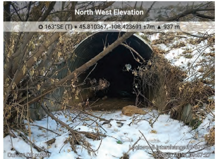
Culvert C9. M.P. 454.74, 102-inch CMP, Outlet
