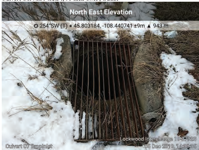
Culvert C7. M.P. 453.77, 24-inch RCP, Drop Inlet
