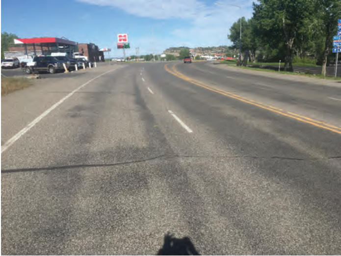
Highway 87 typical transverse cracks and minor rutting, looking northwest. Cracks have been sealed.
