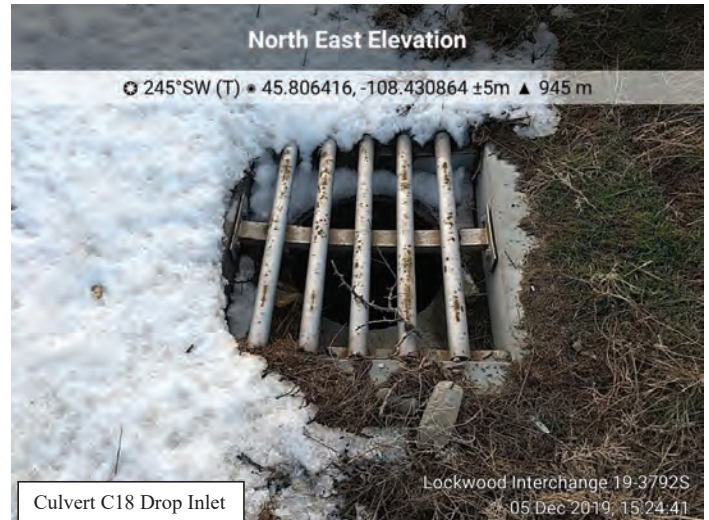
Culvert C18. M.P. 454.29, 24-inch RCP, Drop Inlet
