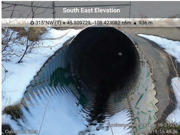
Culvert C9. M.P. 454.75, 102-inch CMP, Inlet
