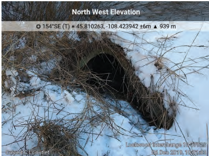
Culvert C17. M.P. 454.73, 24-inch RCP, Outlet
