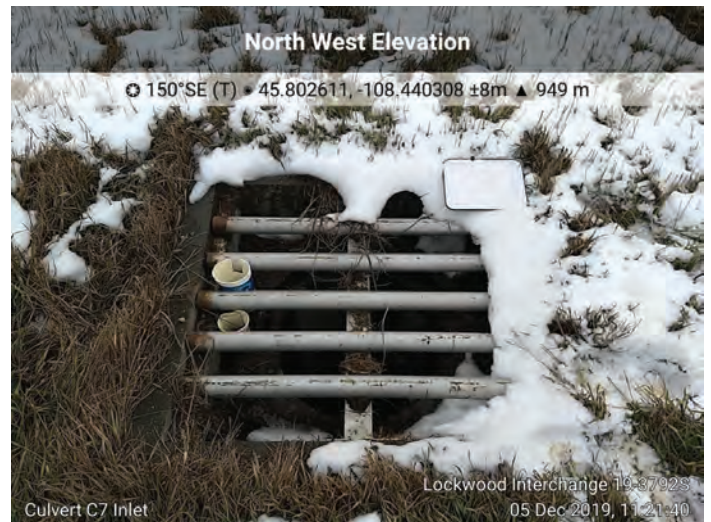
Culvert C7. M.P. 453.77, 24-inch RCP, Drop Inlet
