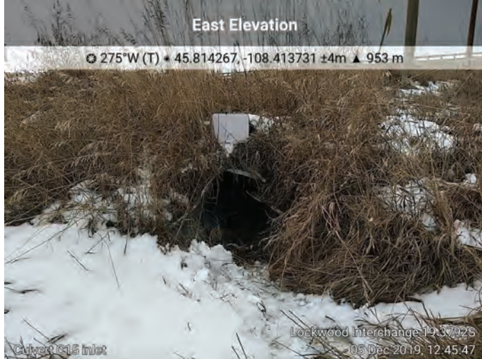
Culvert C15. M.P. 455.29, 24-inch CMP, Inlet
