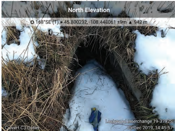
Culvert C3. M.P. 453.36, 24-inch RCP, Outlet
