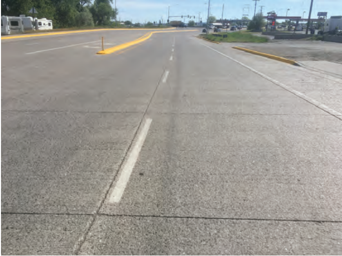
Highway 87 typical PCCP worn surface, and some minor infrequent broken edges.
