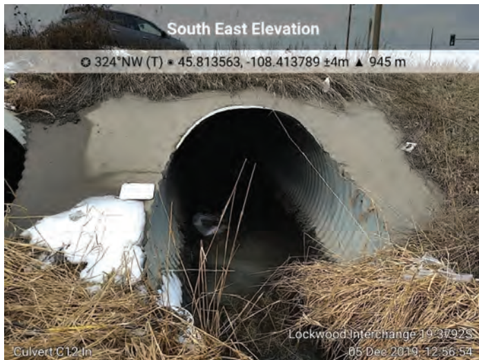
Culvert C12. M.P. 455.27, 72-inch CMP, Inlet
