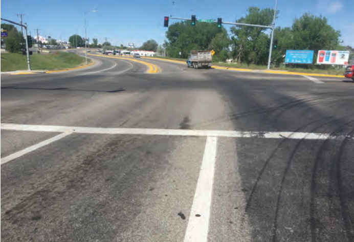
Intersection of Highway 87 and North Frontage Road, looking west. Minor patches and reflecting at the joints, but otherwise in good shape.
