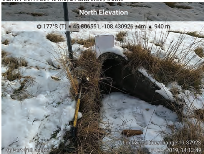
Culvert C18. M.P. 453.29, 24-inch RCP, Outlet
