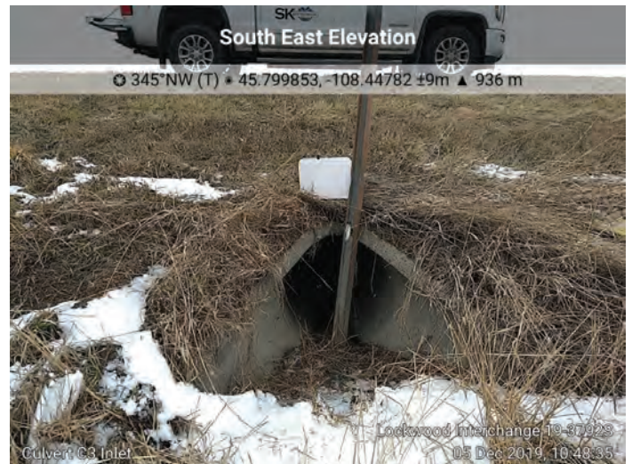
Culvert C3. M.P. 453.36, 24-inch RCP, Inlet
