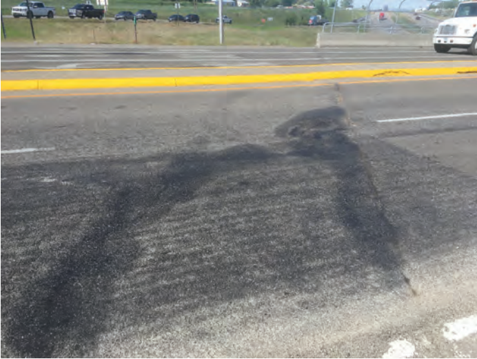
Highway 87 Lockwood Interchange south bridge end pavement distress, looking west. Rutting, transverse cracks, patches, and block cracking.
