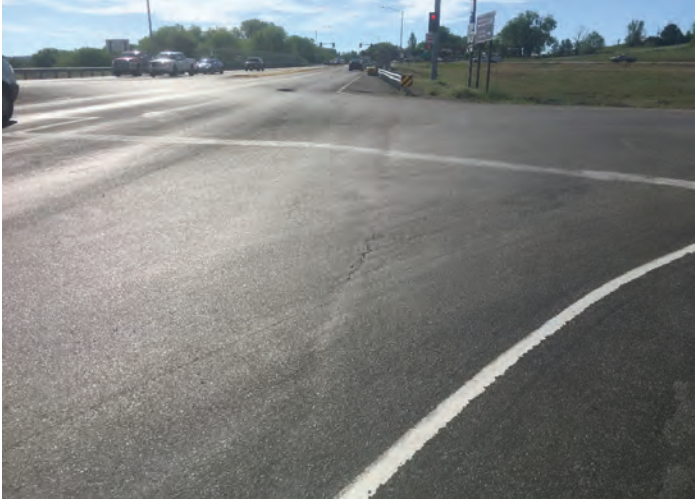
Highway 87 turn to I-90 westbound on ramp. Joint cracking observed across lane.
