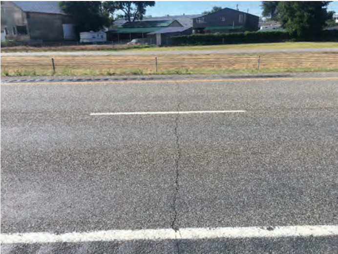
I-90 eastbound and westbound mainline, typical transverse crack.
