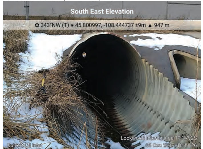
Culvert C4. M.P. 453.53, 90-inch CMP, Inlet
