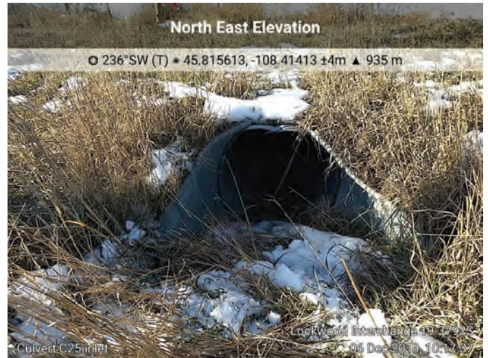
Culvert C25. M.P. 455.39, 24-inch CMP, Inlet
