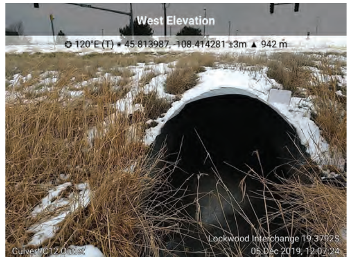
Culvert C12. M.P. 455.25, 72-inch CMP, Outlet
