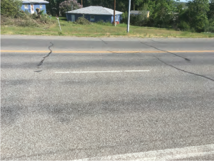
Highway 87 typical transverse cracks and minor rutting, looking east. Cracks have been sealed.
