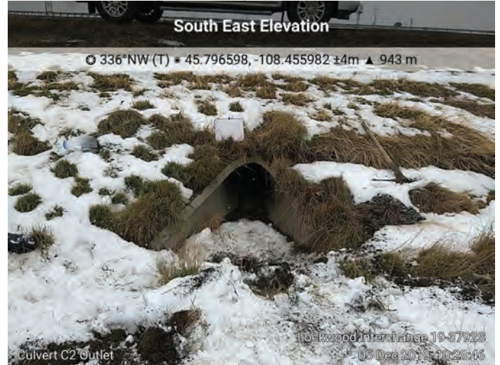
Culvert C2. M.P. 452.90, 24-inch RCP, Outlet
