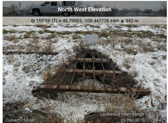
Culvert C5. M.P. 453.55, 24-inch RCP, Inlet
