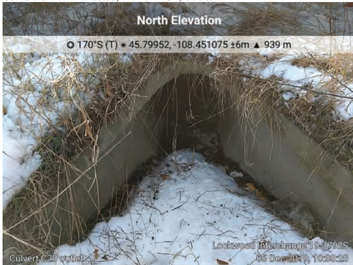
Culvert C20. M.P. 453.21, 24-inch RCP, Outlet
