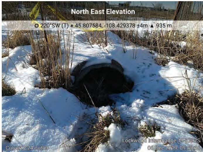
Culvert C24. M.P. 454.36, 24-inch RCP, Outlet
