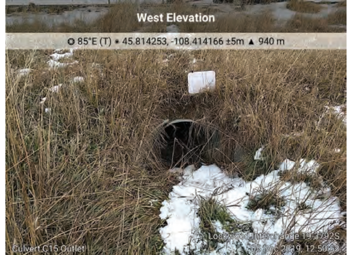
Culvert C15. M.P. 455.27, 24-inch CMP, Outlet
