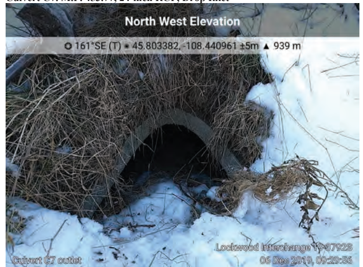
Culvert C7. M.P. 453.77, 24-inch RCP, Outlet
