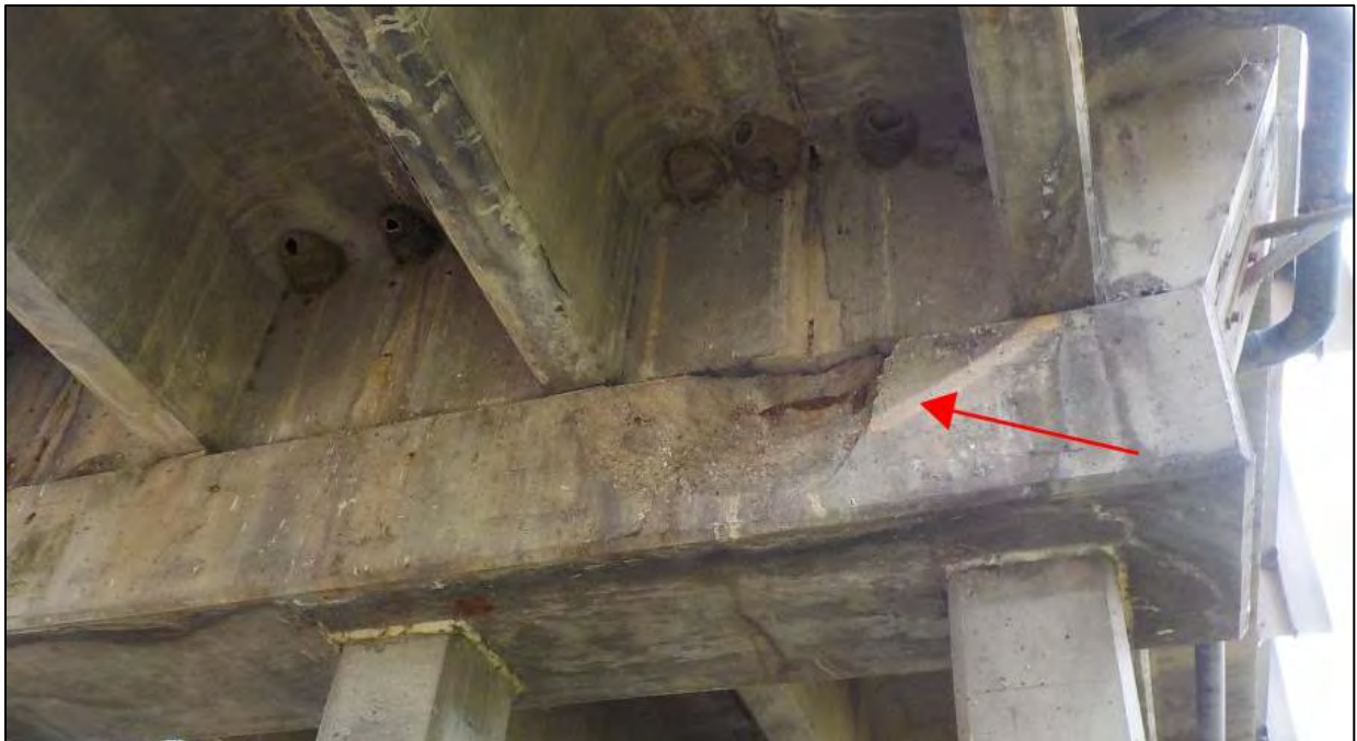
Photo 59: Bent 4 had a 3 ft. wide by 2 ft. high spall with exposed reinforcing steel on the west face of the bent cap. The exposed reinforcing steel had moderate corrosion with negligible section loss
