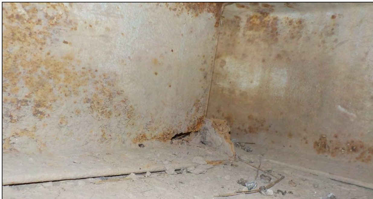
Photo 47: Span 1, Abutment 1, Stringer 7: the stringer web had heavy corrosion and section loss over a 14 in. long by 2 in. high area with a 2 in. long by 1/2 in. high hole center 2 in. from the stringer end
