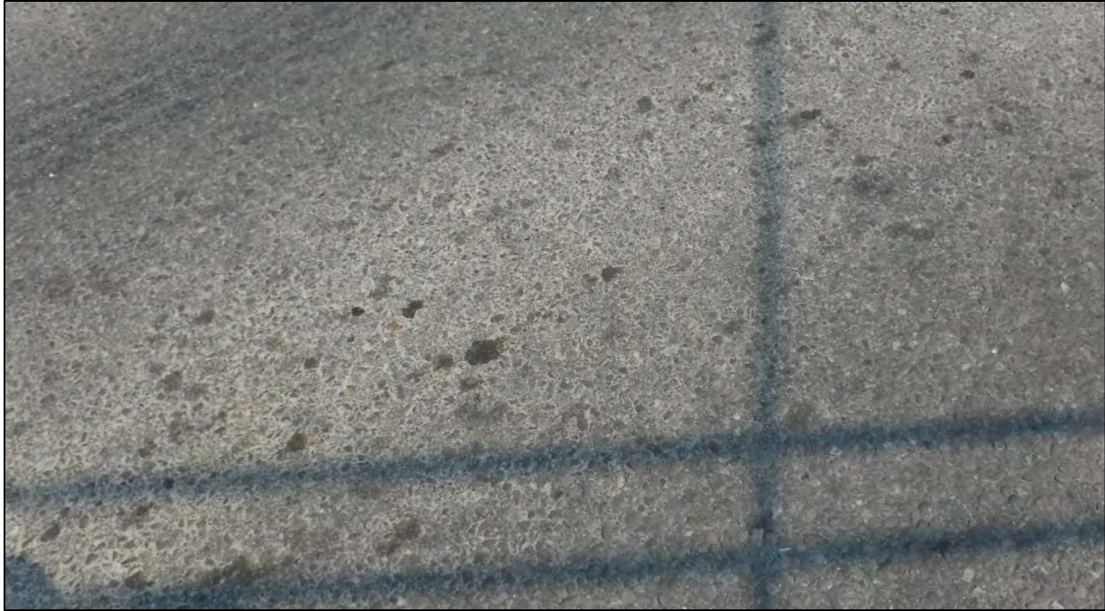
Photo 22: Typical minor wear on Span 1 bituminous overlay
