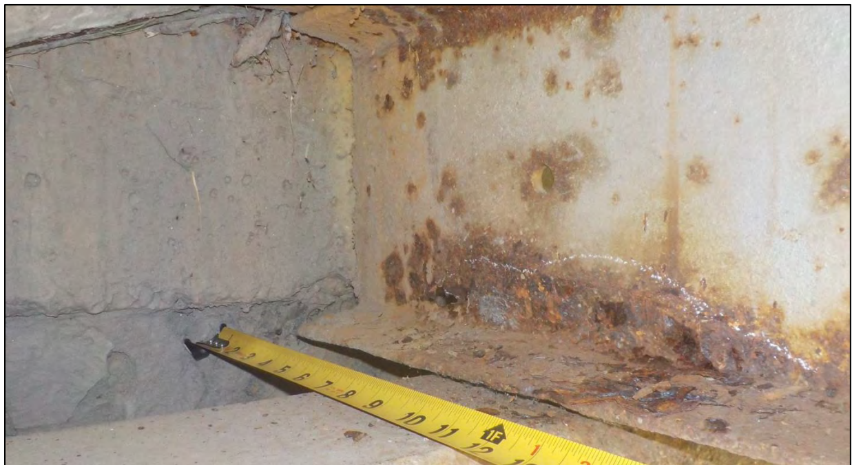
Photo 53: Span 2, Bent 3, Stringer 7: the stringer web had heavy corrosion with up to 50 percent section loss over a 6 in. long by 2 in. high adjacent to the stringer end that had a 1/2 in. diameter hole 6 in. from the stringer end at the web to lower flange interface
