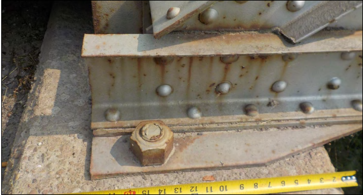
Photo 68: Bent 2, South Truss, Span 2 fixed bearing
