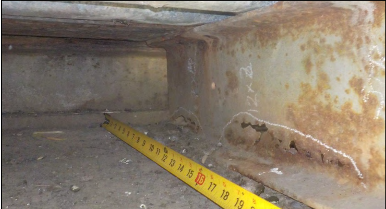
Photo 48: Span 2, Bent 2, Stringer 2: the stringer web had heavy corrosion and section loss with two holes; 7 in. long by 1 in. high and 6 in. long by 2 in. high centered 16 in. from the stringer end
