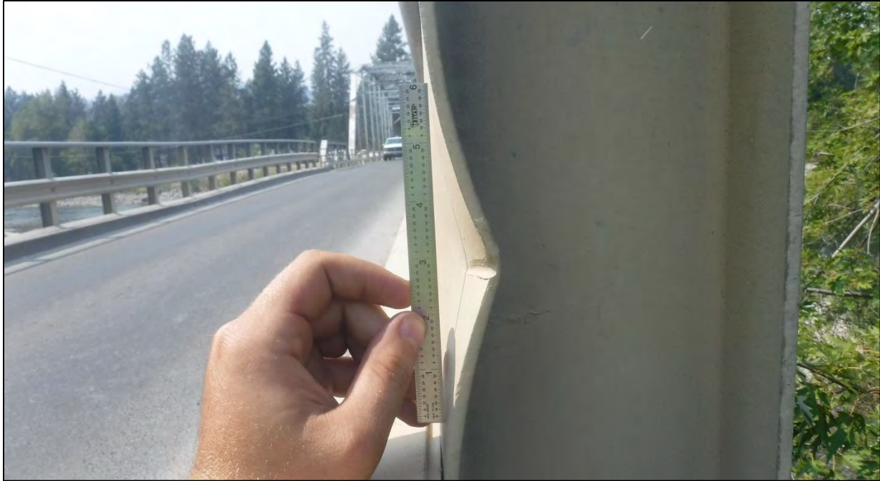
Photo 36: Three vertical members had impact damage that bent the interior flange 3/4 in. over a 6 in. length on the North Rail near the East Approach
