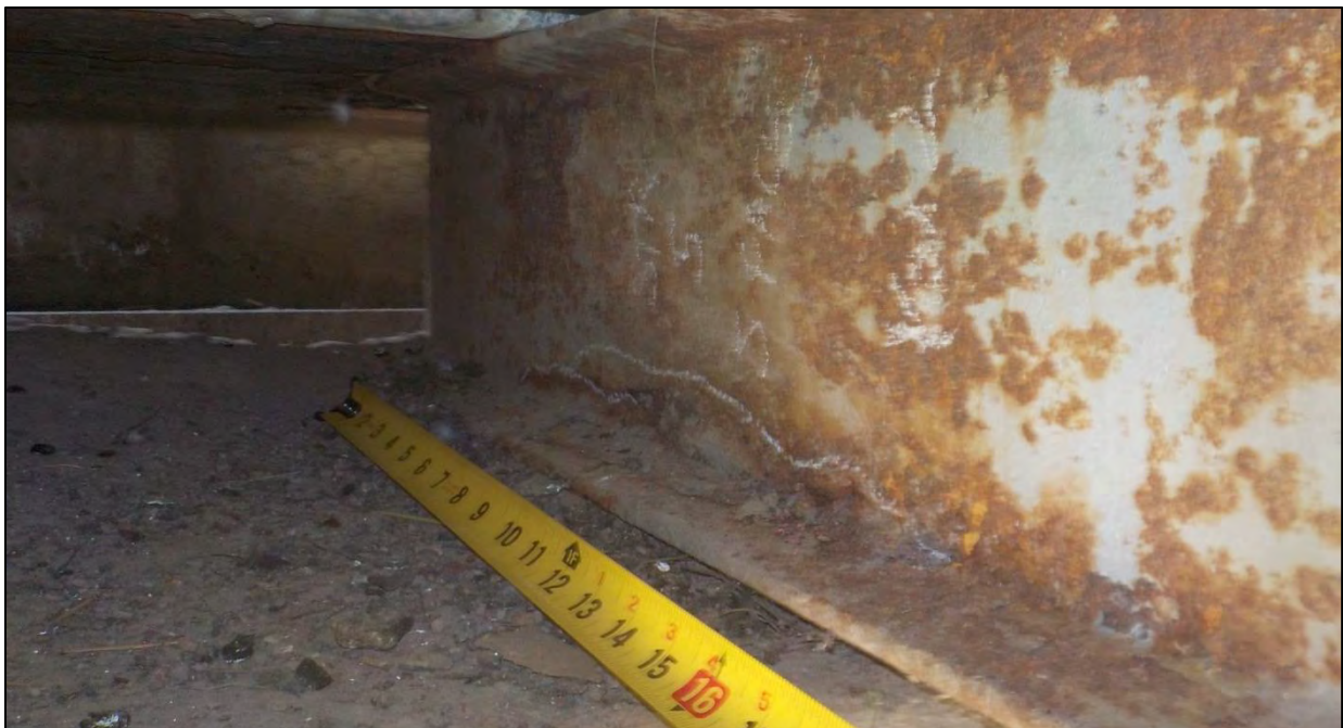
Photo 49: Span 2, Bent 2, Stringer 5: the south face had a 16 in. long by 2 in. tall area of pack rust up to 1/4 in. thick on the bottom of the web located 12 in. from the end of the stringer
