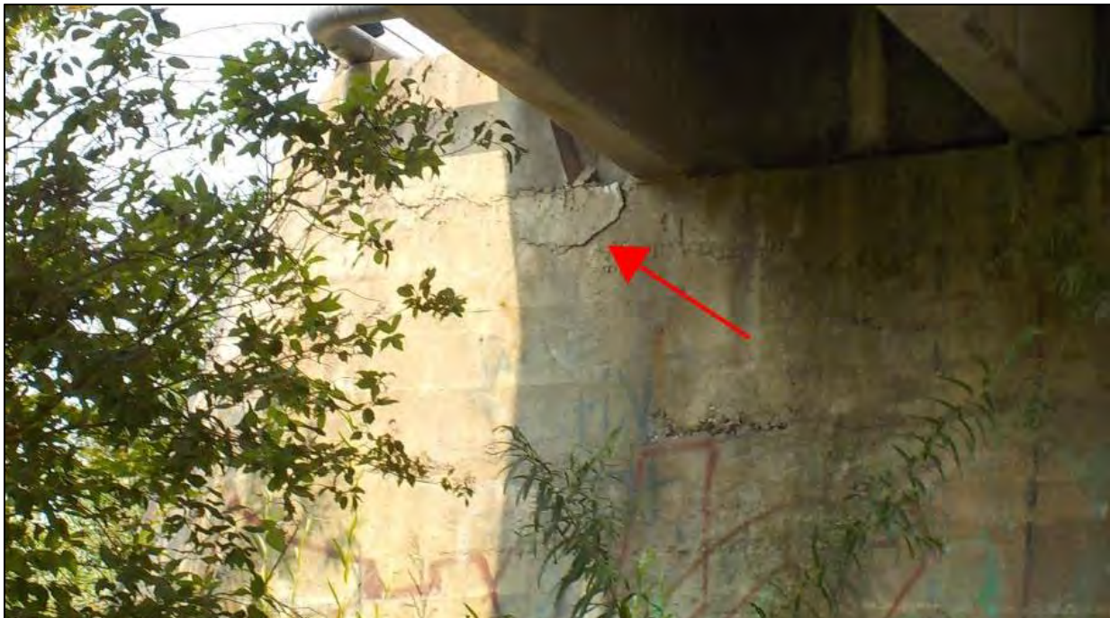
Photo 57: Bent 3 had a 12 in. wide by 10 in. high area of delamination on the top, southeast corner of the bent
