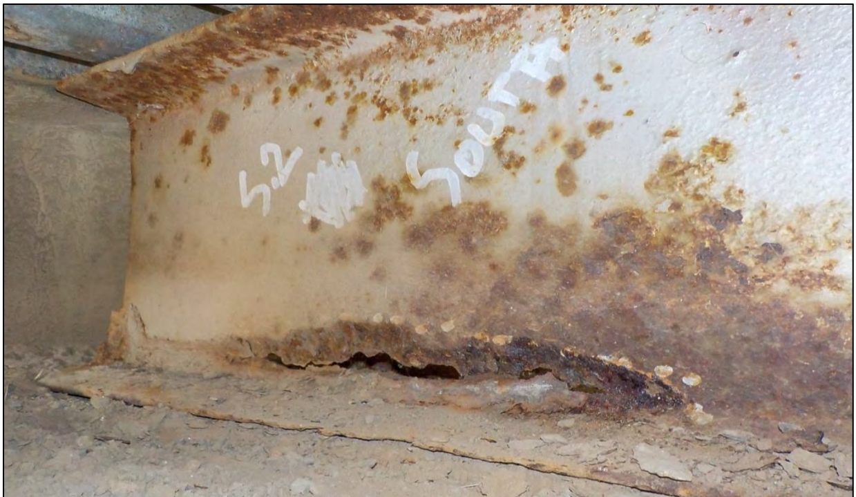
Photo 45: Span 1, Abutment 1, Stringer 2: the stringer web had heavy corrosion and section loss over a 17 in. long by 2 in. high area with a 1 in. diameter hole center 10 in. from the stringer end
