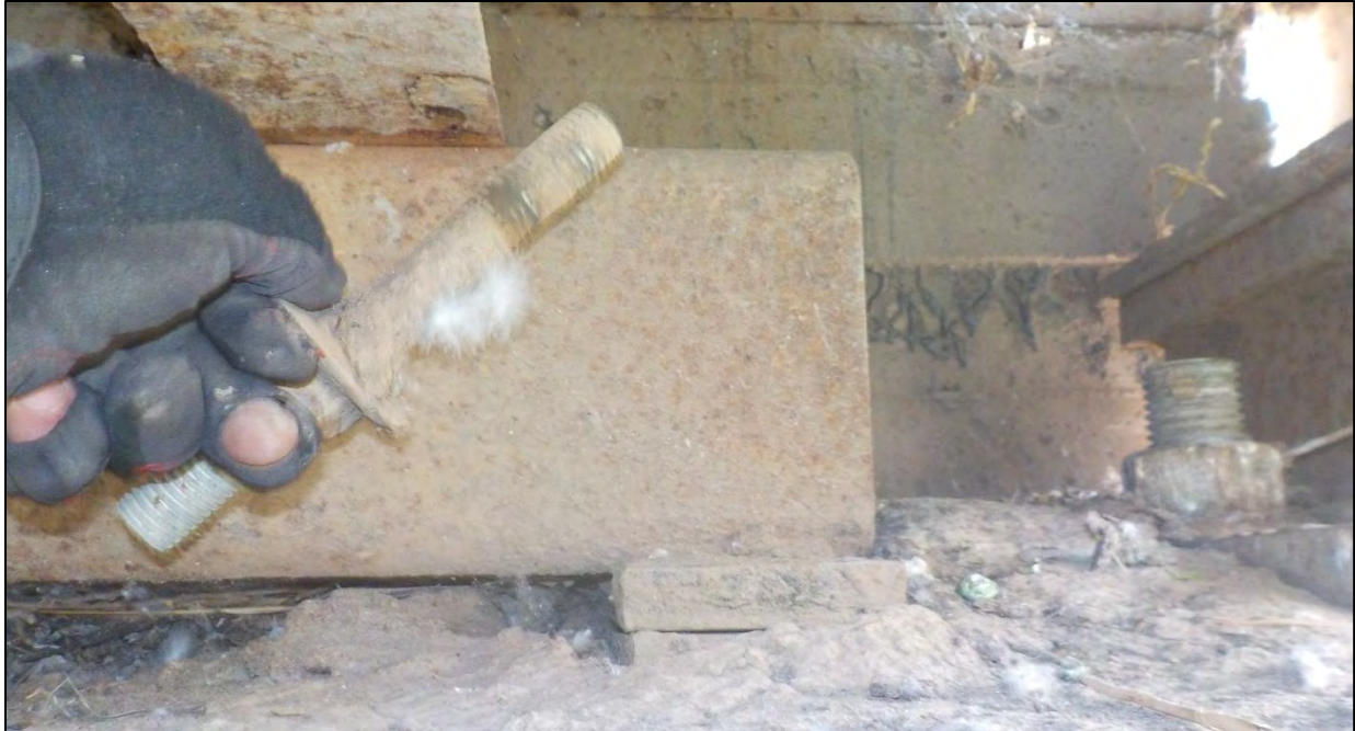
Photo 50: Span 2, Bent 3, All Stringers: the hollow pipe that the stringers were bearing on had vertical movement up to 1/4 in. when vehicles passed. The south anchor rod for the south pipe had failed and this edge of the pipe had movement up to 1/2 in. when vehicles passed
