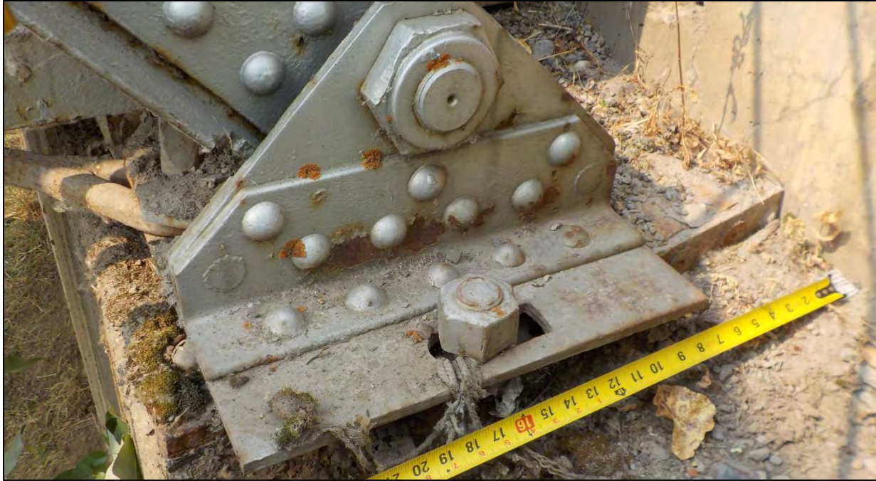
Photo 60: Abutment 1, North Truss roller bearing
