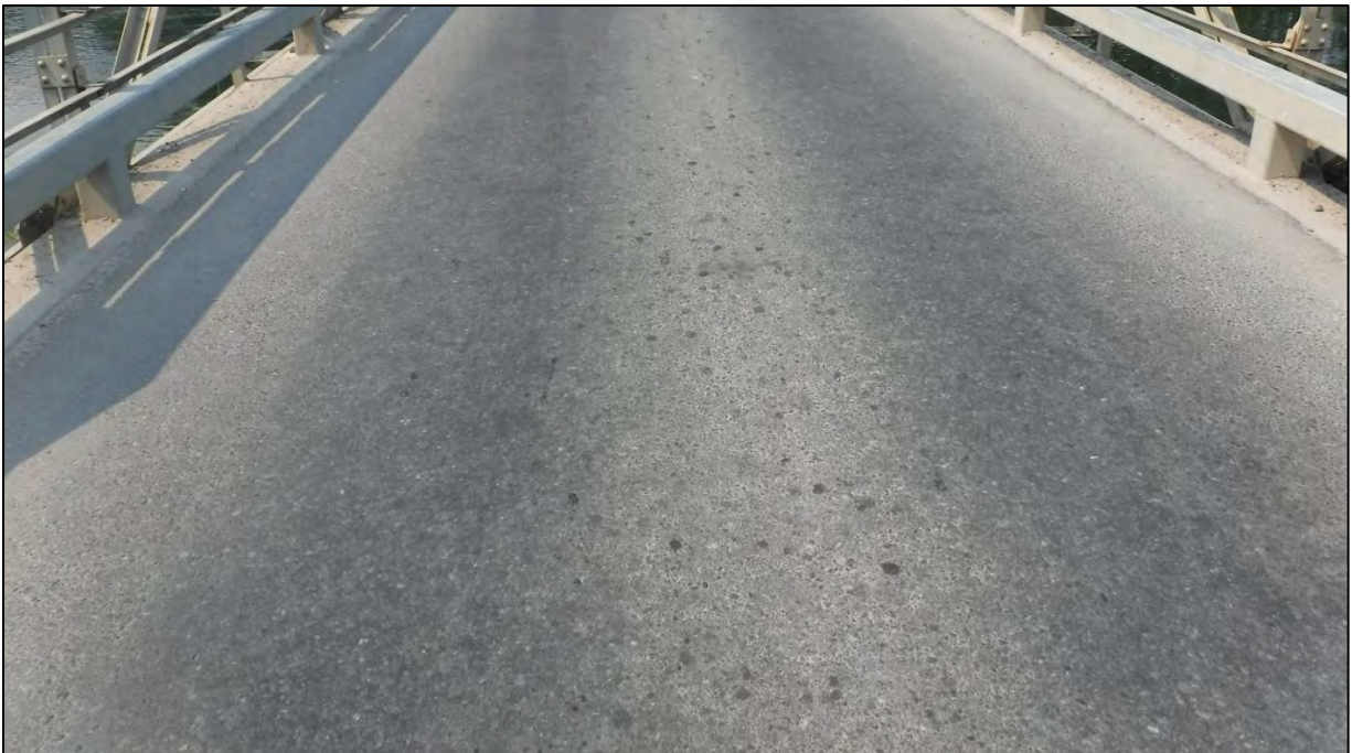
Photo 37: Typical minor wear on Span 2 bituminous overlay
