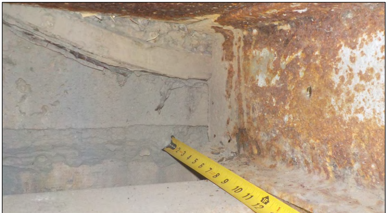
Photo 50: Span 2, Bent 3, All Stringers: the hollow pipe that the stringers were bearing on had vertical movement up to 1/4 in. when vehicles passed. The south anchor rod for the south pipe had failed and this edge of the pipe had movement up to 1/2 in. when vehicles passed
