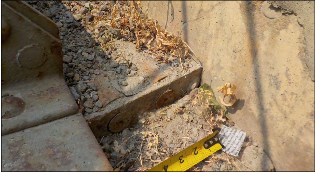
Photo 64: Abutment 1, South Truss roller bearing with the rollers and roller keeper protruding out from underneath the bearing and resting against the abutment backwall
