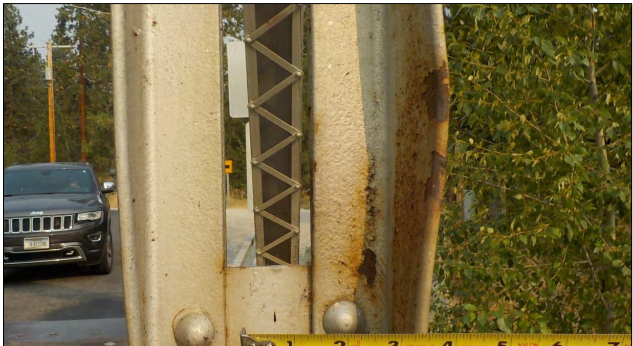
Photo 71: Span 1, North Truss, Vertical U1-L1: the exterior flange of the vertical was bent 1 in. to the north due to impact damage approximately 5 ft. above the bridge deck
