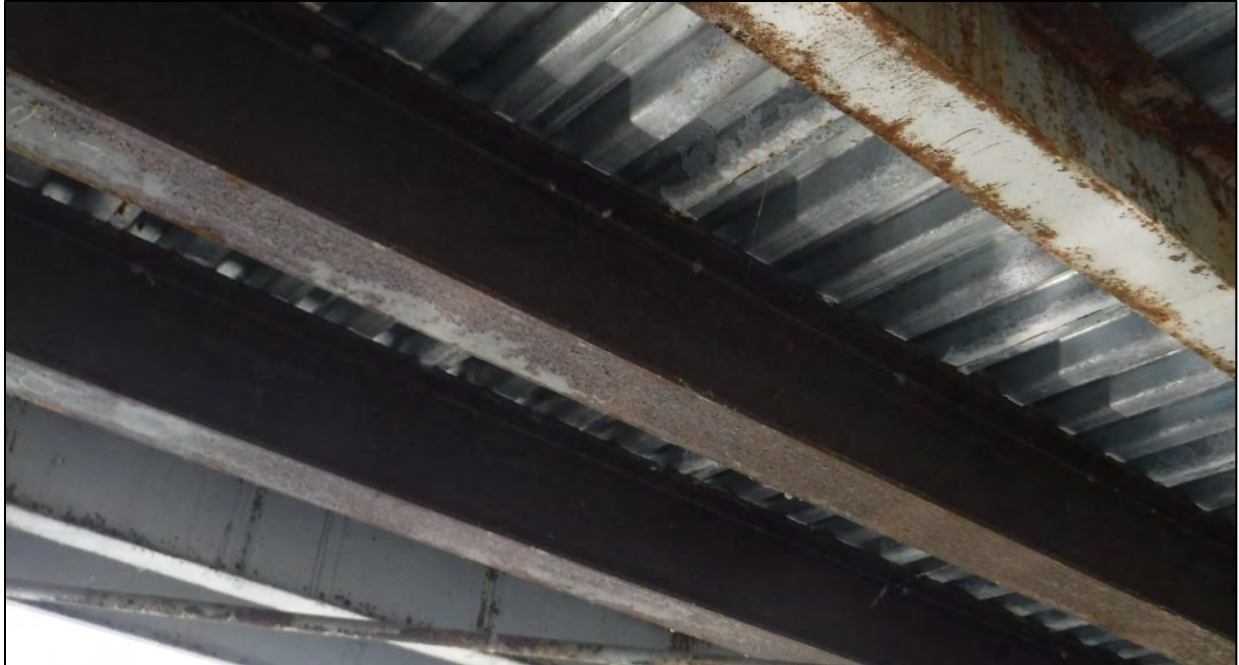
Photo 44: Typical unpainted stringers with minor to moderate corrosion and negligible section loss
