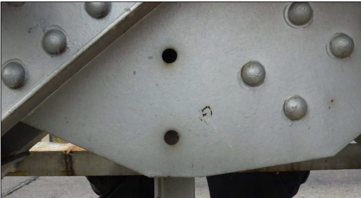
Photo 75: Span 2, North Truss, Gusset Plate U1': the exterior gusset plate had two misdrilled 3/4 in. diameter holes
