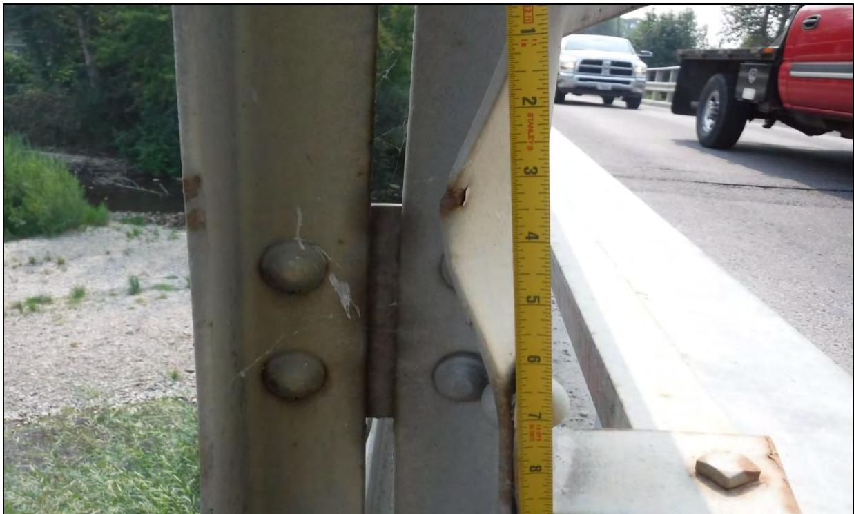
Photo 73: Span 2, North Truss, Vertical L2'-U2': the interior flange of the vertical was bent 1 in. over a 6 in. length due to impact damage
