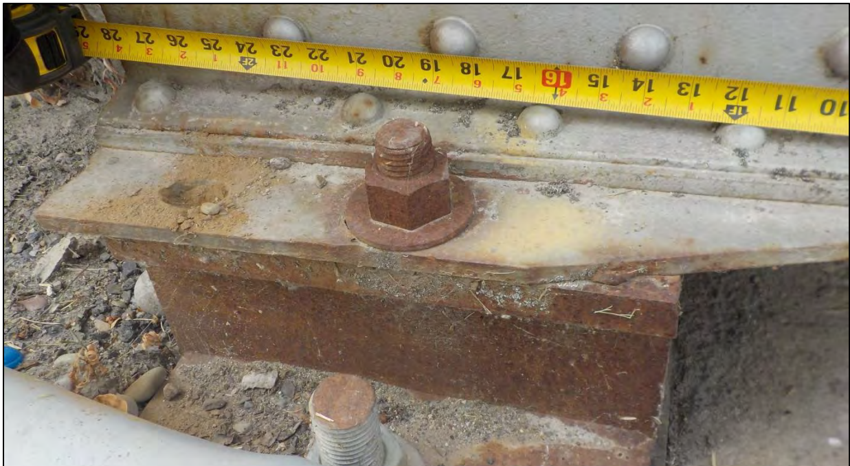
Photo 69: Bent 3, North Truss, Span 2 slider bearing
