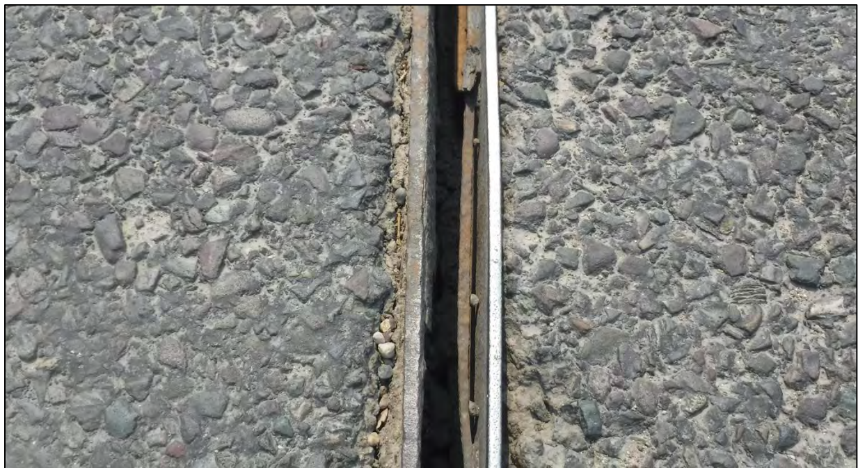
Photo 41: Joint 3 over Bent 3 with seal deterioration which was typical over 90 percent of the length
