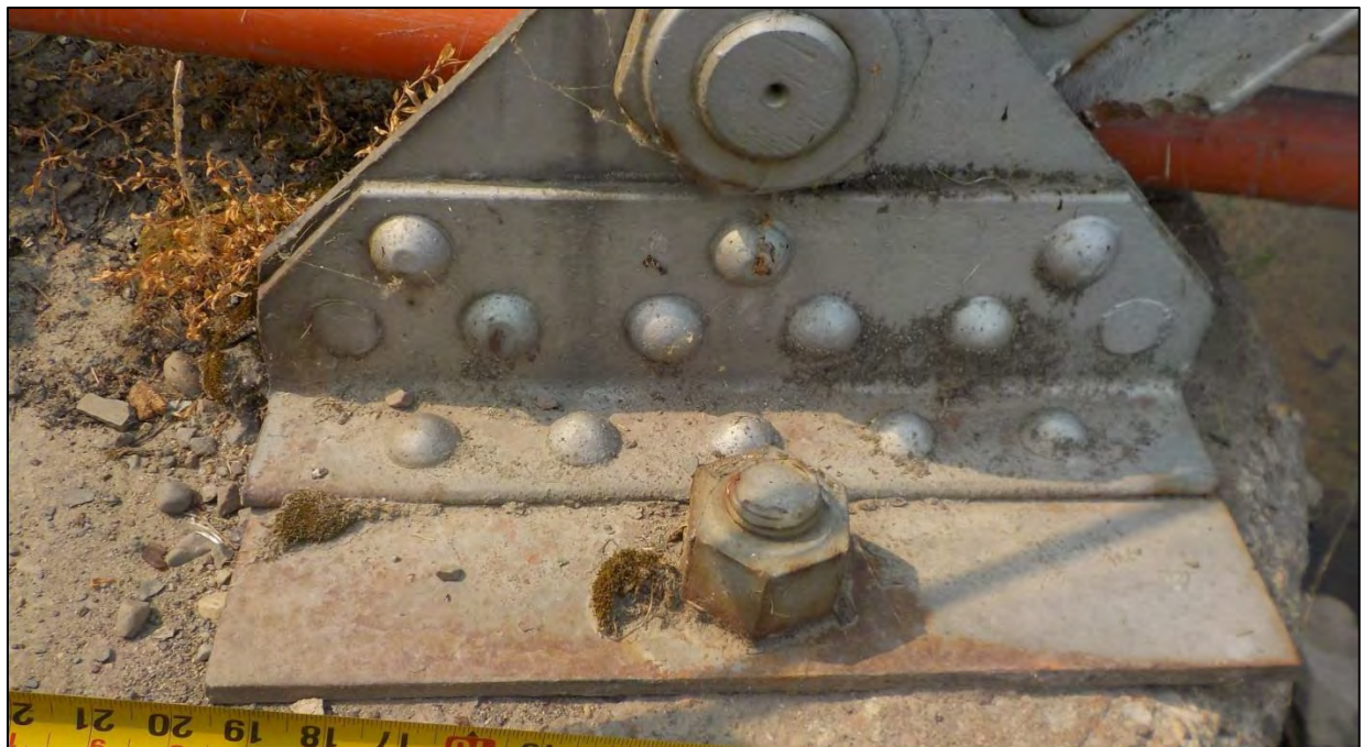
Photo 65: Bent 2, North Truss, Span 1 fixed bearing
