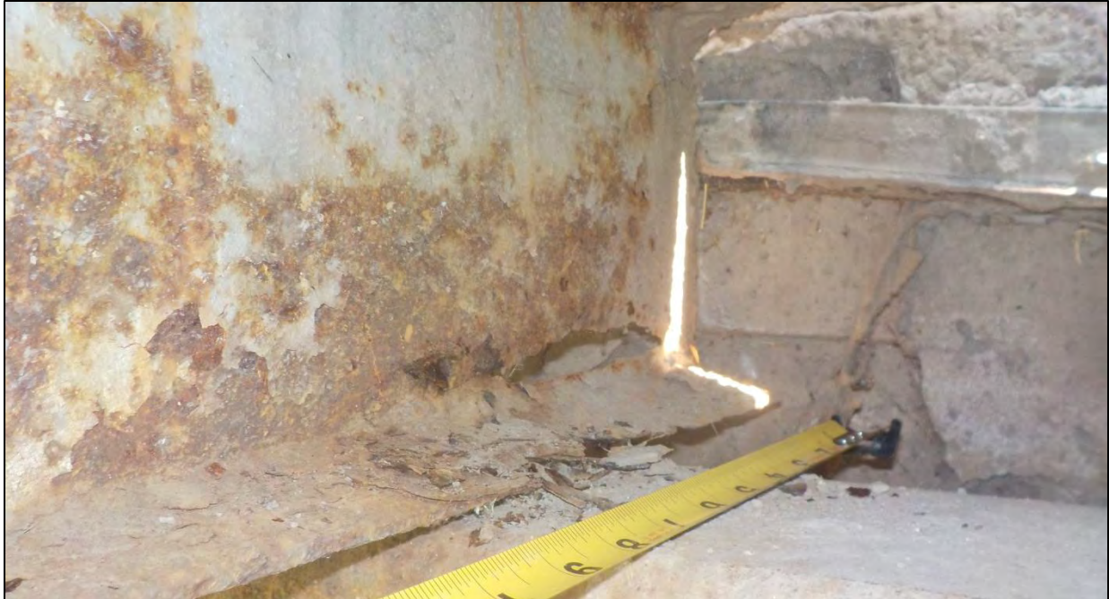
Photo 52: Span 2, Bent 3, Stringer 4: the stringer web had heavy corrosion and section loss with a 5 in. long by 1 in. high through hole near the stringer end. The bottom flange was knife edges in this area
