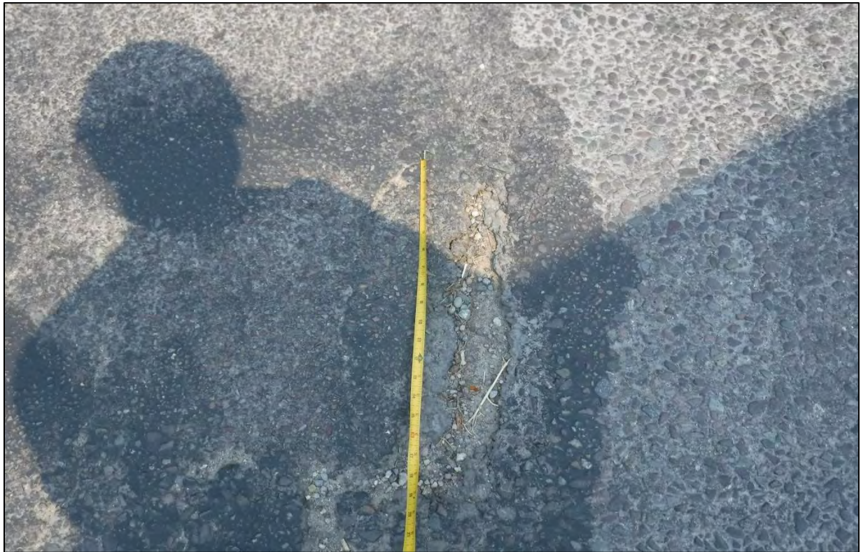
Photo 23: Typical minor wear on Span 1 bituminous overlay
