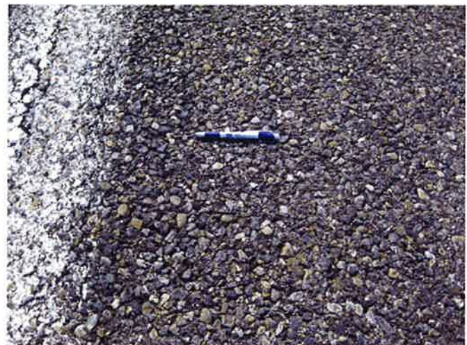
R-1, Surface detail with raveling
