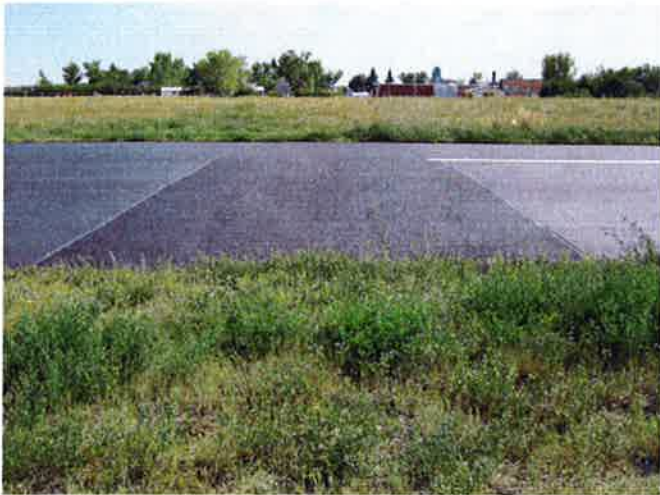
R-1 , Surface detail with patching 2
