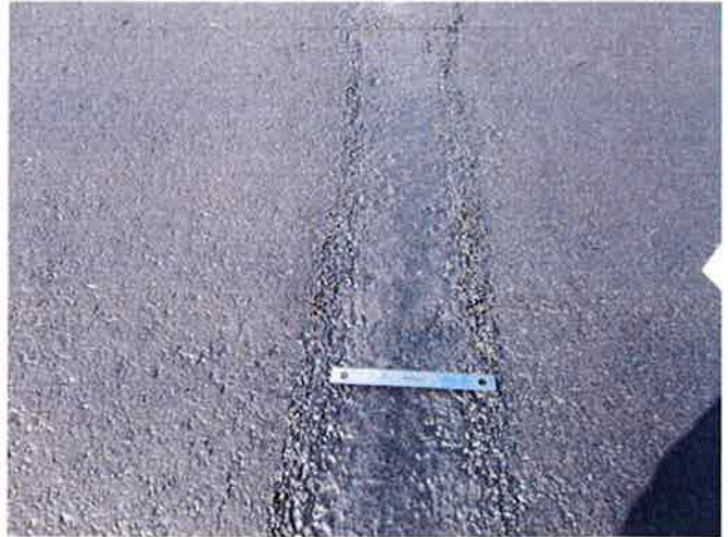
R-1 , Surface detail with patch
