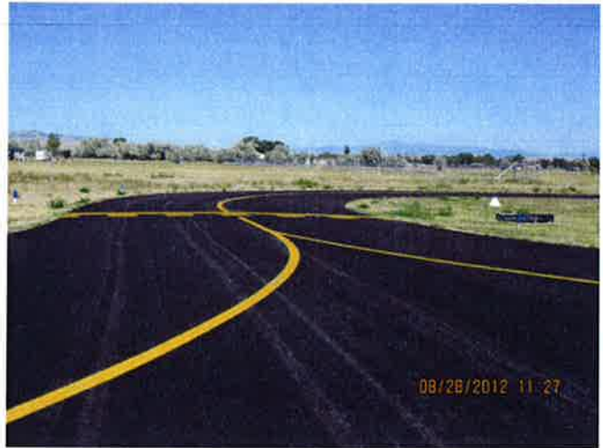
T-2, Taxiway overview
