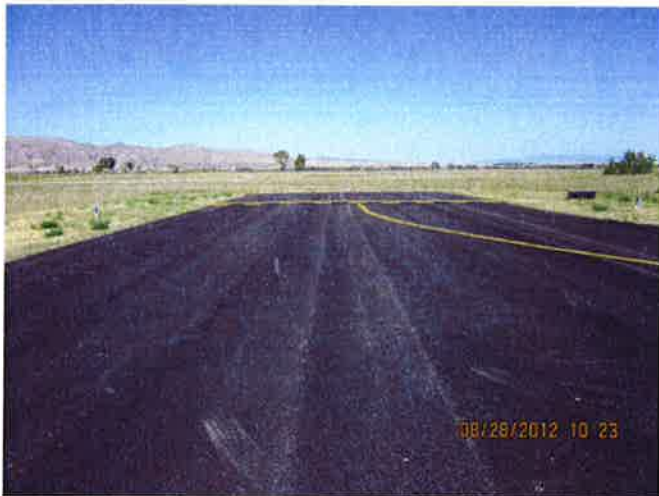
T-2, Turnaround overview
