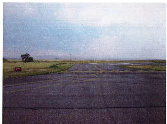
T-2, Taxiway Overview 2
