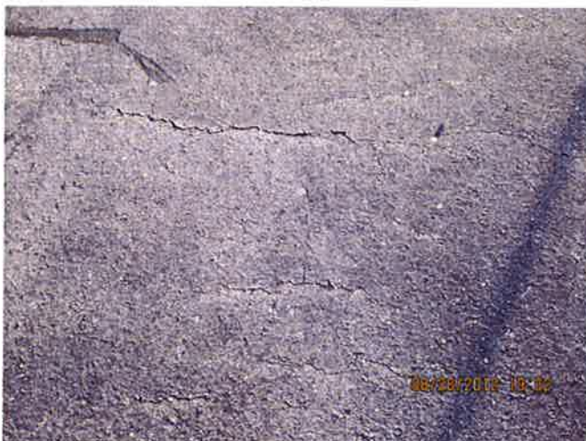
T-2, Hangar area surface detail with cracking
