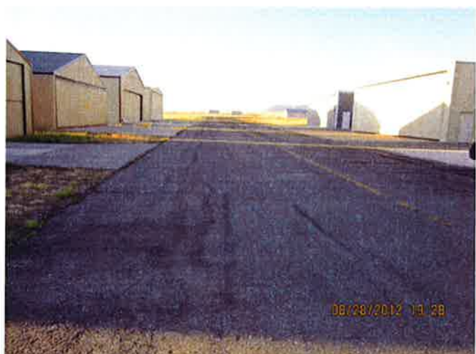
T-2, Overview hangar area
